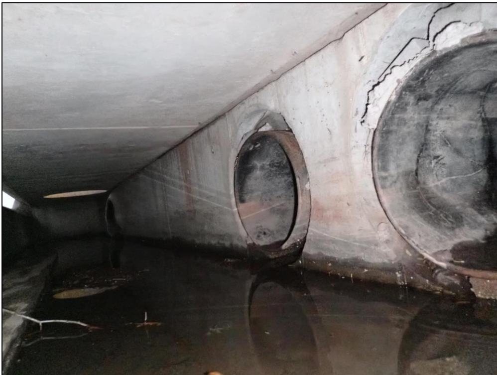
4576: Inside Outfall Structure 11, looking upstream along the Western principal spillway pipe. Damage to outlet pipe or structure, pipe connections are not sealed (Routine Maintenance Needed).
