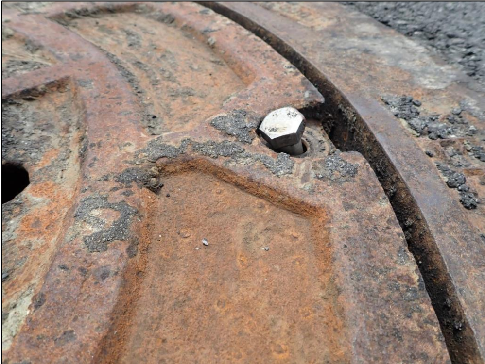
5099: Close-up of Manhole 6. Inadequate access to complete a thorough inspection, bent bolt (Routine Maintenance Needed).
