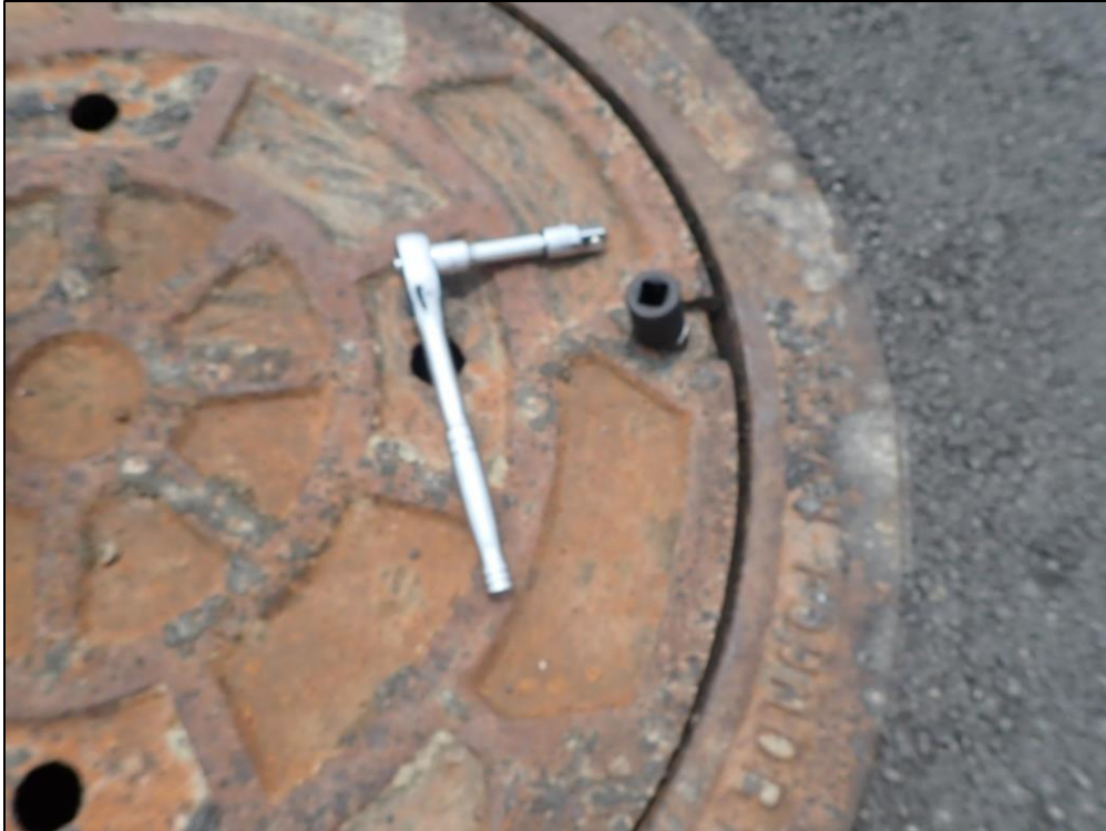
5100: Close-up of Manhole 6. Inadequate access to complete a thorough inspection, bent bolt (Routine Maintenance Needed).
