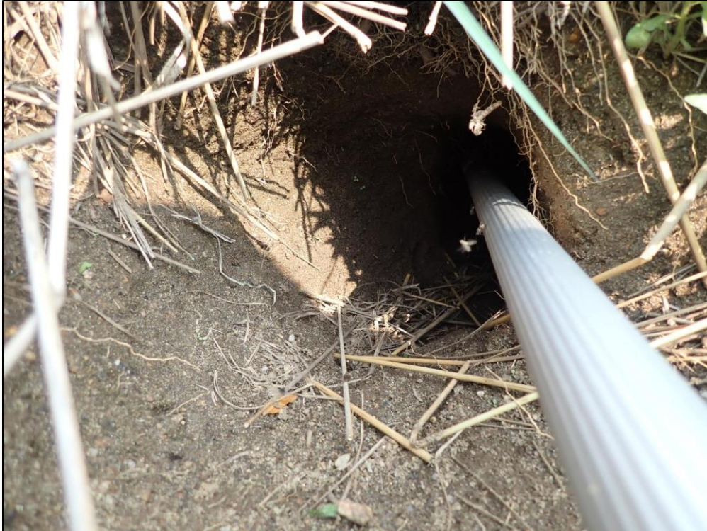
5016: Close-up of the Animal Hole. Evidence of nuisance animals (Routine Maintenance Needed).
