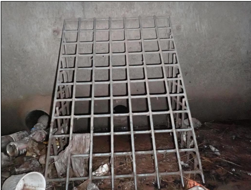
4566: Inside the upstream end of Control Structure 12, looking toward the low-flow orifice. Buildup of trash, debris, and sediment (Monitor).
