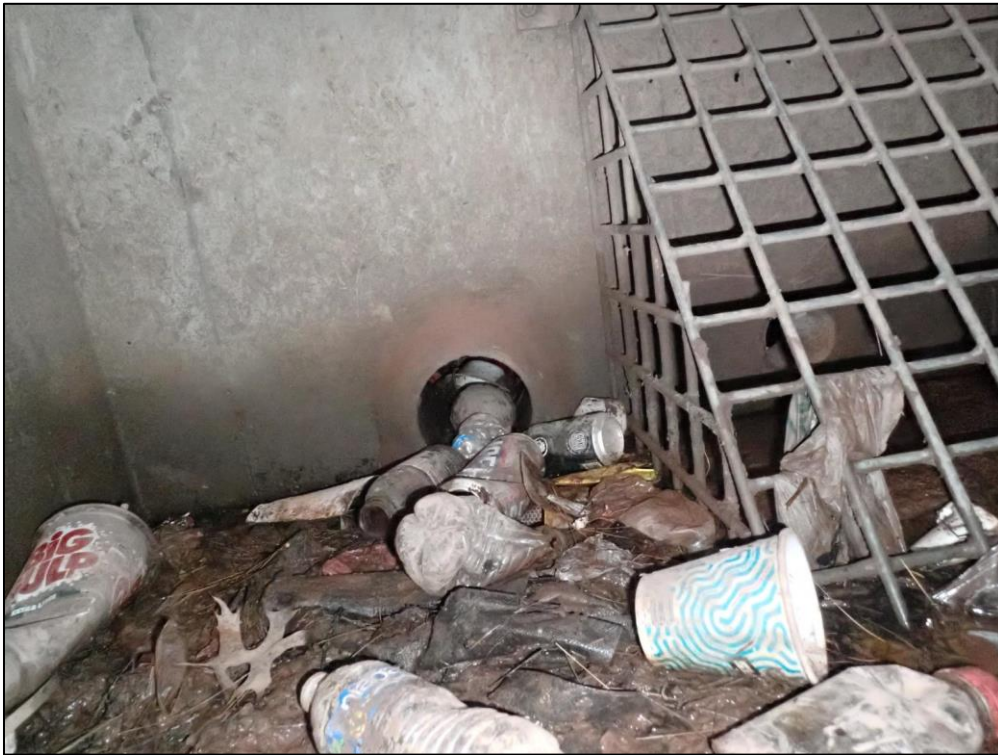
4567: Inside the upstream end of Control Structure 12, looking toward the dewatering valve orifice. Buildup of trash, debris, and sediment (Monitor).
