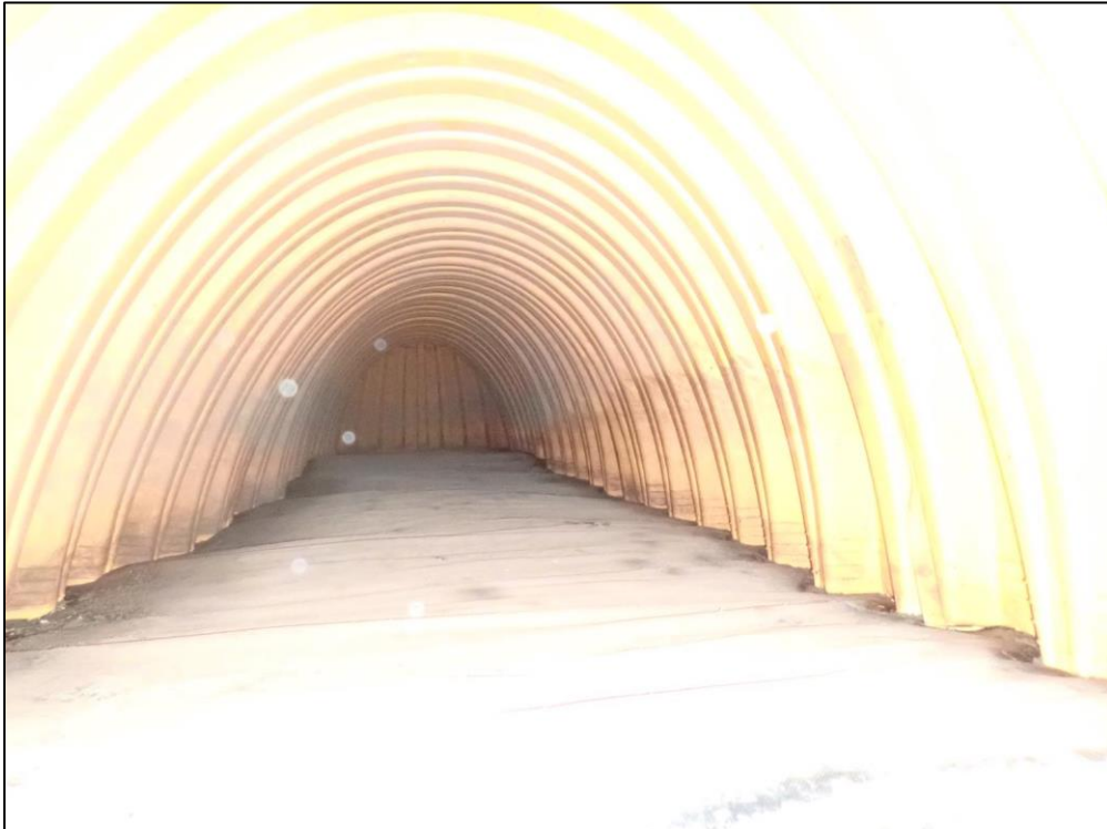
4516: Inside Inspection Port 1, looking downstream along the Southern Isolator Row.
