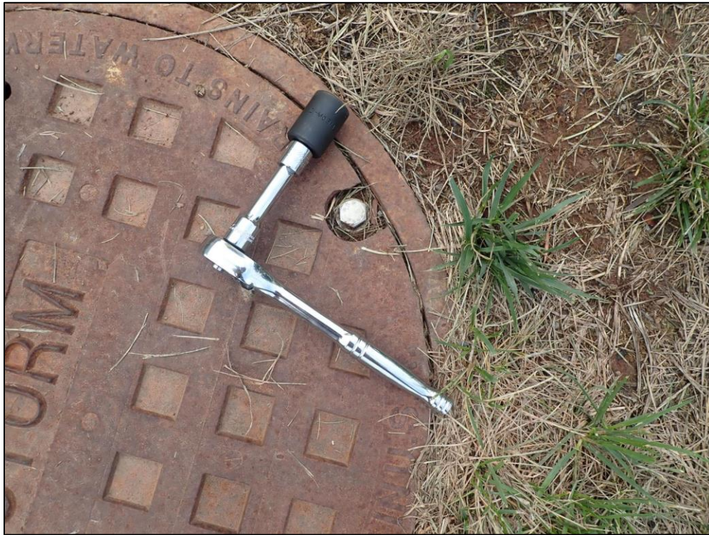
4569: Close-up of the downstream end of Control Structure 12. Inadequate access to complete a thorough inspection; one of the two bolts was stuck (Routine Maintenance Needed).
