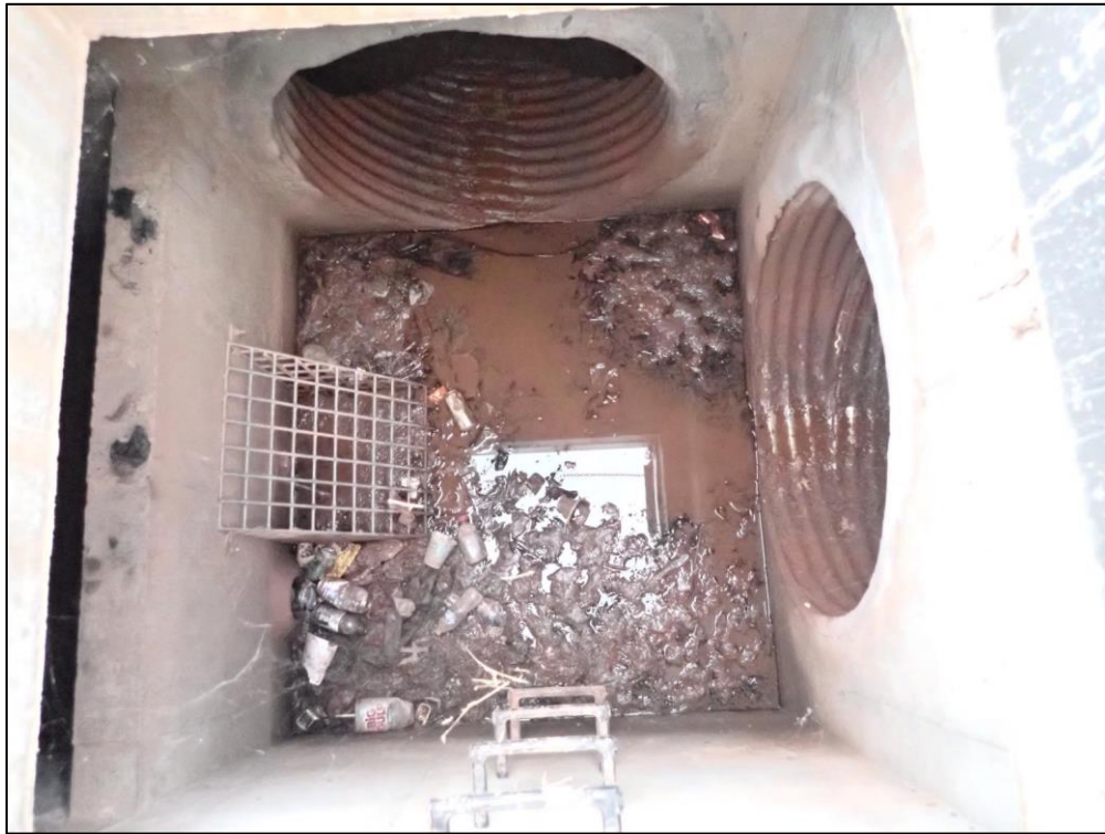
4561: Inside the upstream end of Control Structure 12. Buildup of trash, debris, and sediment (Monitor).
