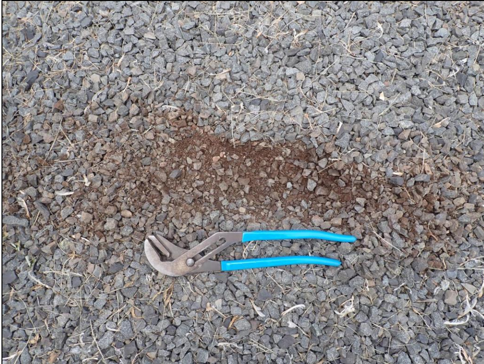
4758: Close-up showing the Gravel Detail. Evidence of clogging (Immediate Repair Needed).
