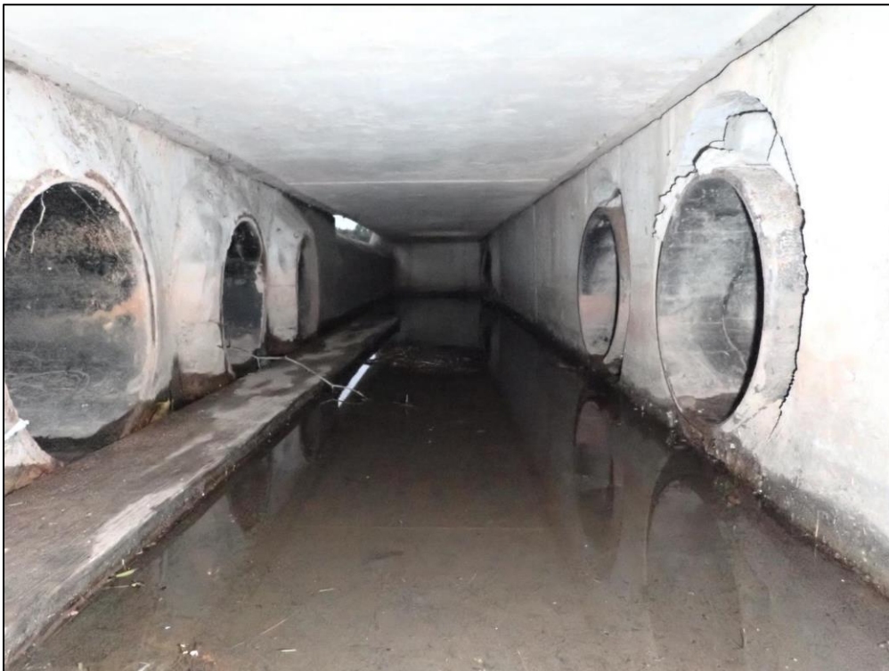
4572: Inside Outfall Structure 11, looking South. Damage to outlet pipe or structure, pipe connections are not sealed (Routine Maintenance Needed).
