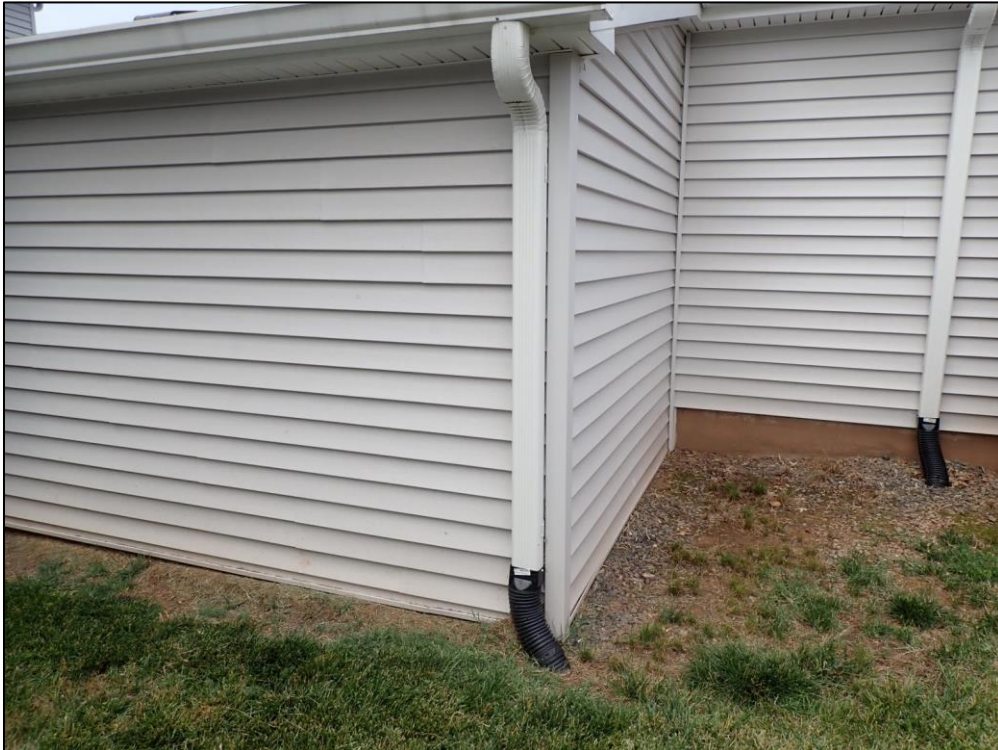
4759: Overall view of Downspout 1, piped underground toward the trench.
