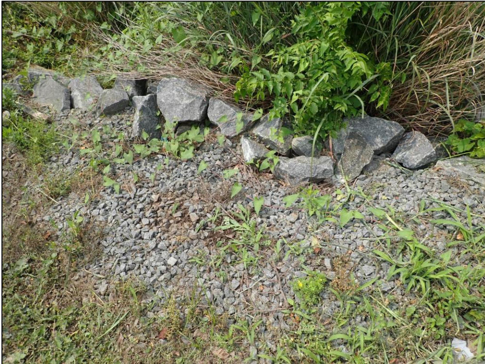
5003: Close-up of the Check dam. Buildup of sediment and vegetation (Routine Maintenance Needed).
