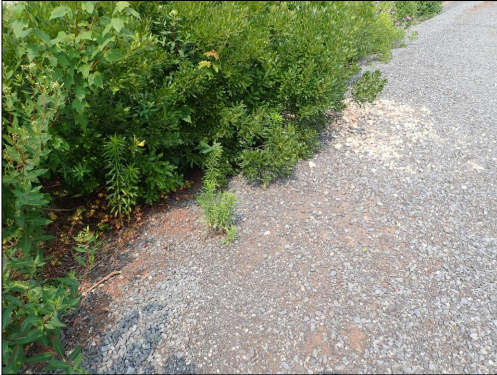
4998: Overall view of the Gravel Diaphragm. Buildup of sediment and vegetation (Routine Maintenance Needed).
