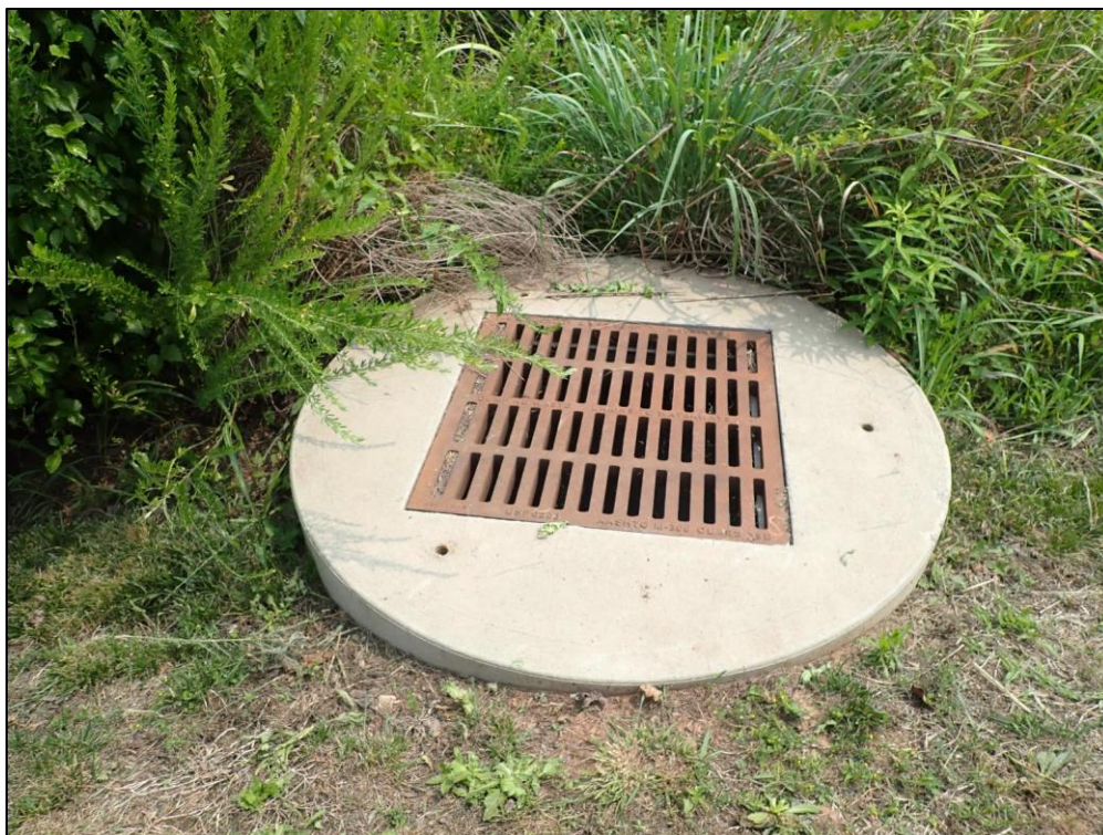
5042: Top of Control Structure 2.
