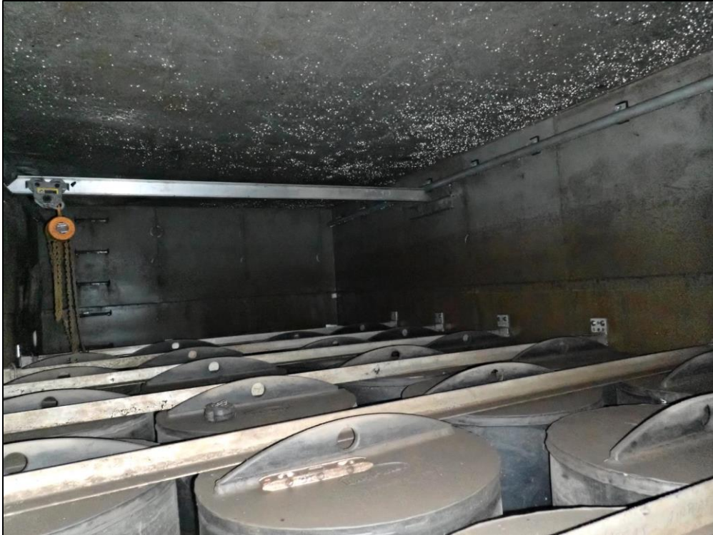
5090: Inside the downstream end of Cartridge Chamber 84, looking toward the filter cartridges.
