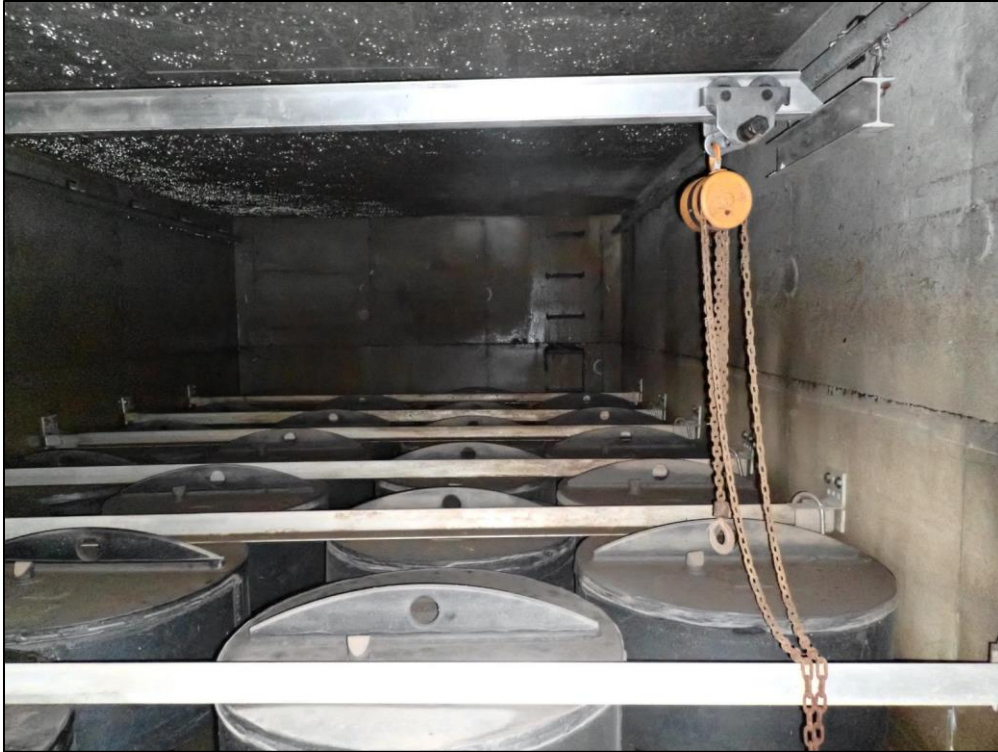
5086: Inside the upstream end of Cartridge Chamber 84, looking toward the filter cartridges.
