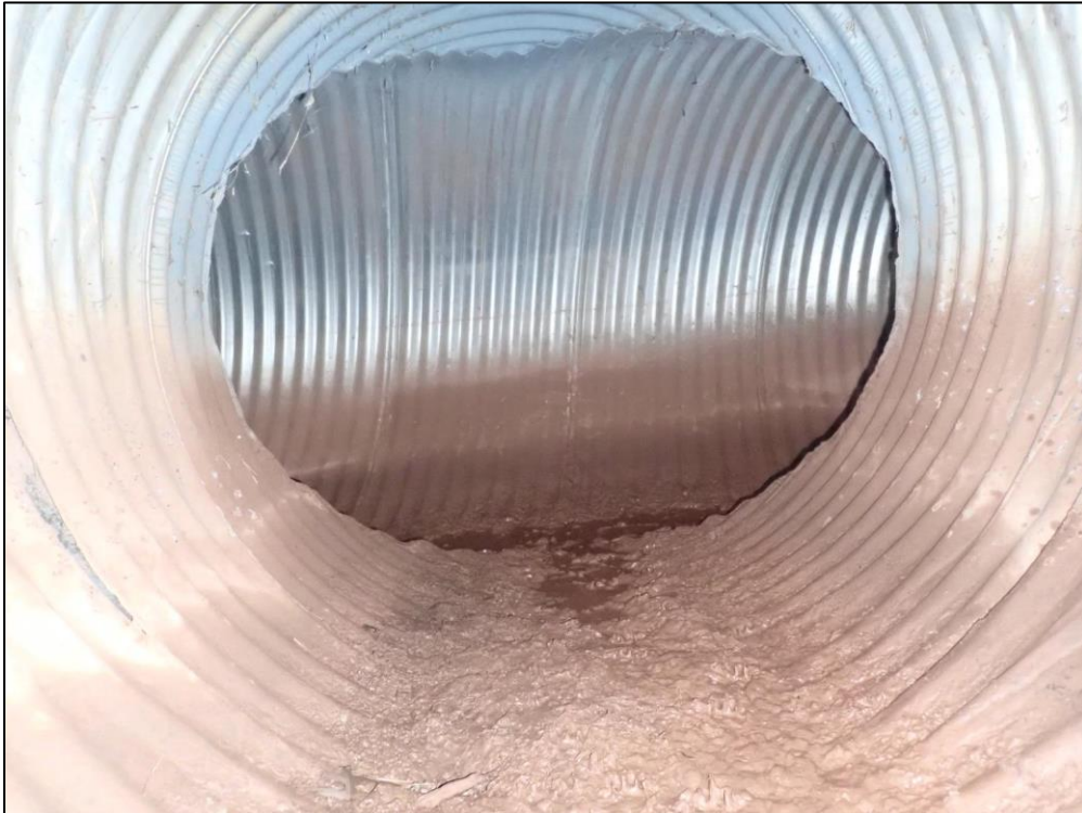
4552: Inside Manhole 1, looking upstream toward the Southern detention pipe joint. Buildup of trash, debris, and sediment (Monitor).
