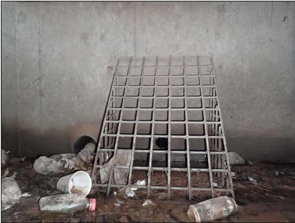
4565: Inside the upstream end of Control Structure 12, looking toward the trash rack. Buildup of trash, debris, and sediment (Monitor).
