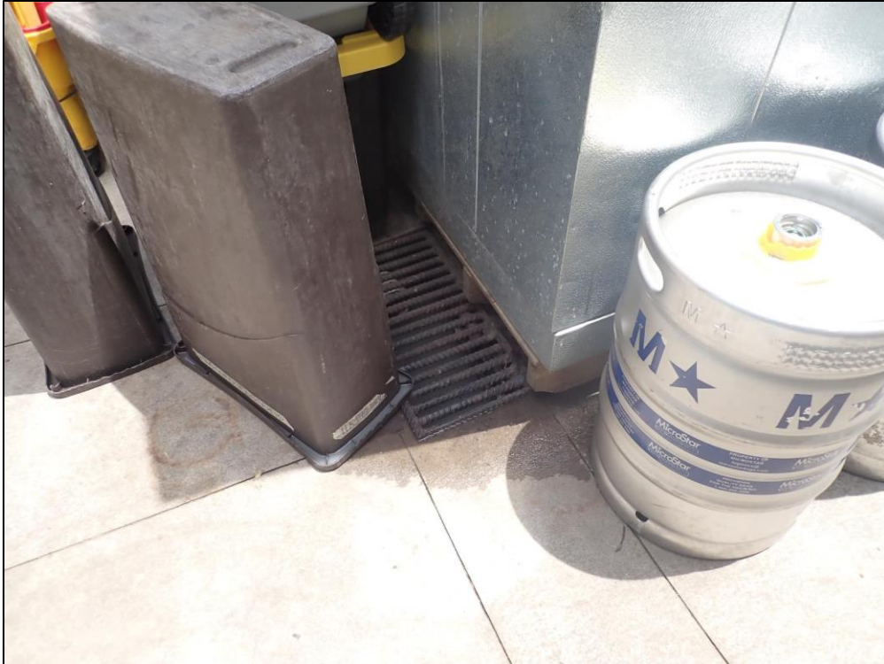
4502: Top of Sidewalk Drain. Surrounding drainage area trash/debris/Unauthorized substances that might affect the facility. (Immediate Repair Needed).
