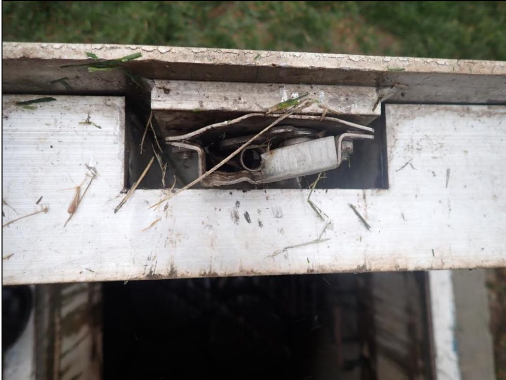
4525: Close-up of the Cartridge Bay access door. Damage to inlet pipe or structure, Broken Bilco door lock (Immediate Repair Needed).
