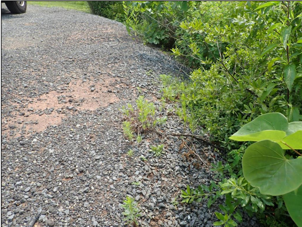
4999: Overall view of the Gravel Diaphragm. Evidence of erosion or bare spots (Routine Maintenance Needed).
