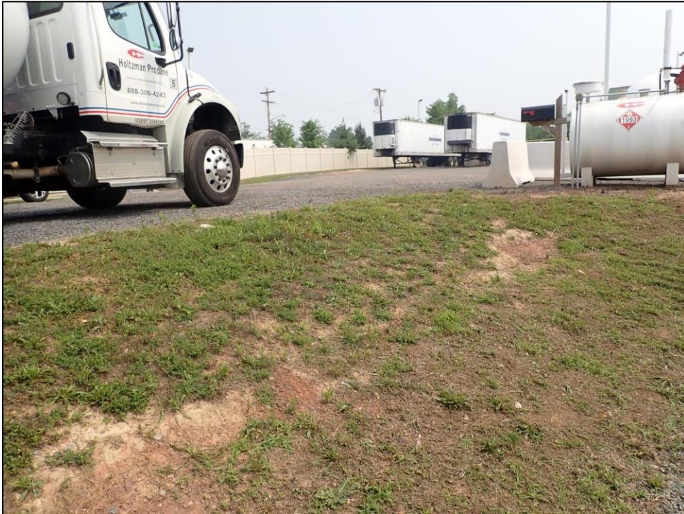
5009: Overall view of the overland inflow area, looking North. Evidence of erosion or bare spots (Routine Maintenance Needed).
