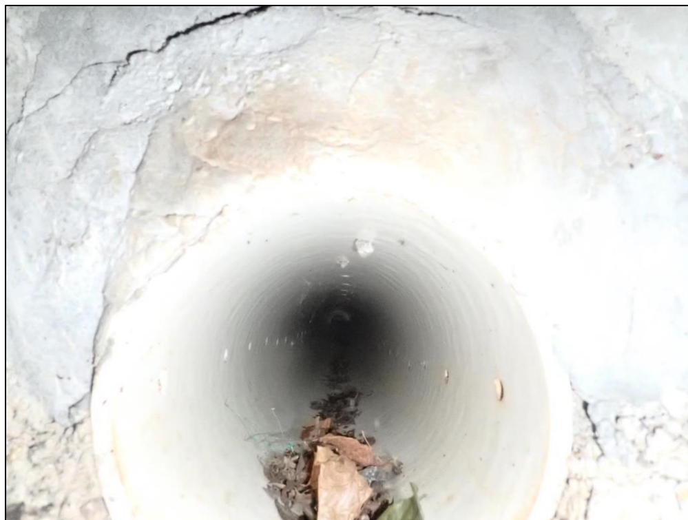
5044: Inside Control Structure 2, looking upstream along the underdrain.
