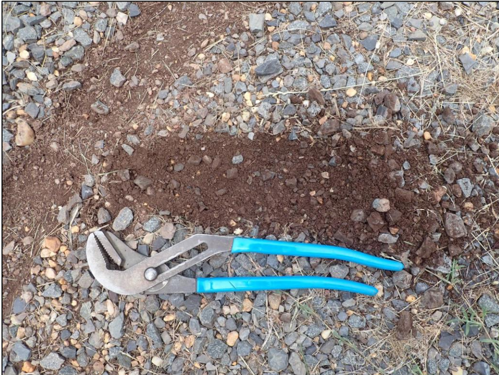
4757: Close-up showing the Gravel Detail. Evidence of clogging (Immediate Repair Needed).
