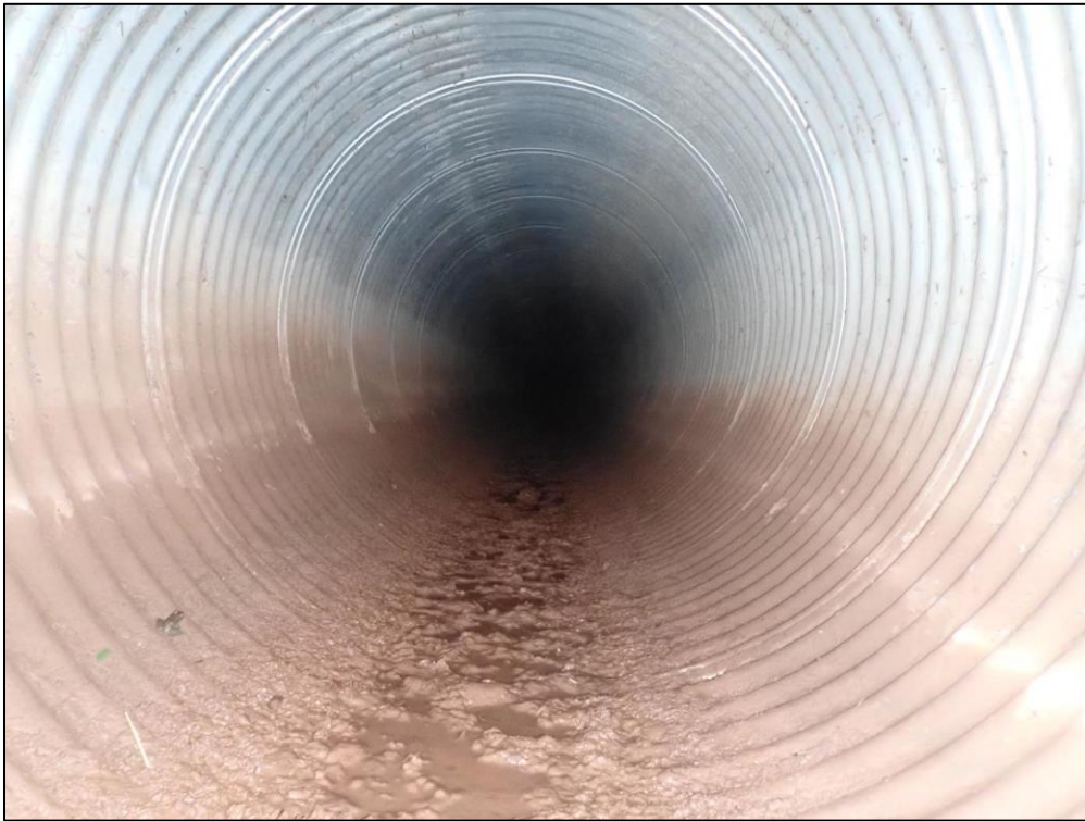
4553: Inside Manhole 1, looking downstream along the middle detention pipe. Buildup of trash, debris, and sediment (Monitor).
