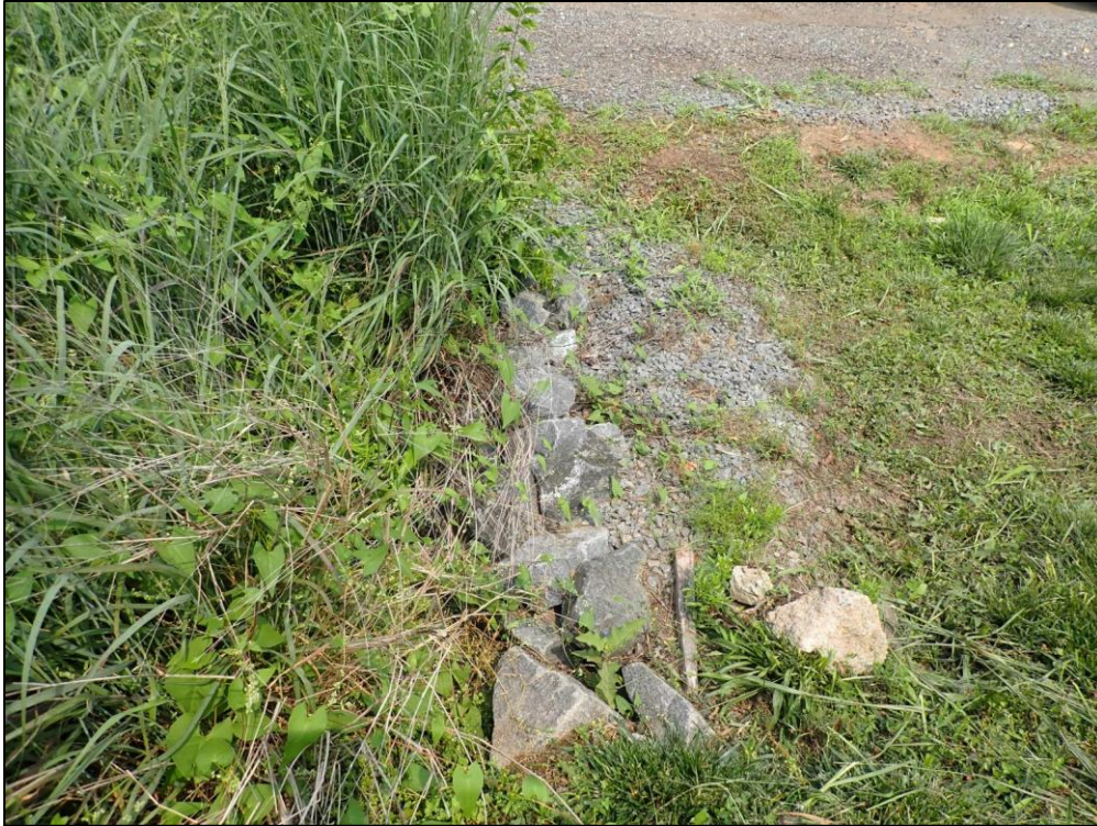
5002: Overall view of the Check Dam. Buildup of sediment and vegetation (Routine Maintenance Needed).
