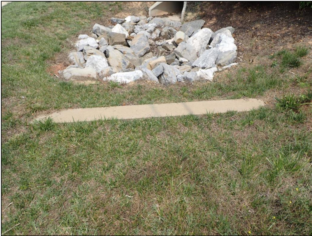
5050: Looking upstream toward the Level Spreader.
