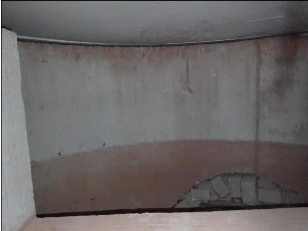
4543: Inside Control Structure 3, looking toward detention. Damage to outlet pipe or structure, pipe connections are not sealed (Routine Maintenance Needed).
