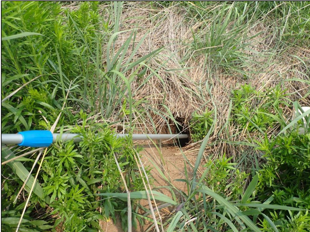
5015: Overall view of the Animal Hole. Evidence of nuisance animals (Routine Maintenance Needed).
