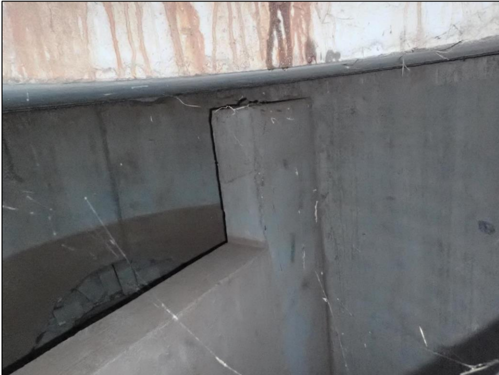
4538: Inside Control Structure 3, looking towards the weir. Damage to outlet pipe or structure, pipe connections are not sealed (Routine Maintenance Needed).
