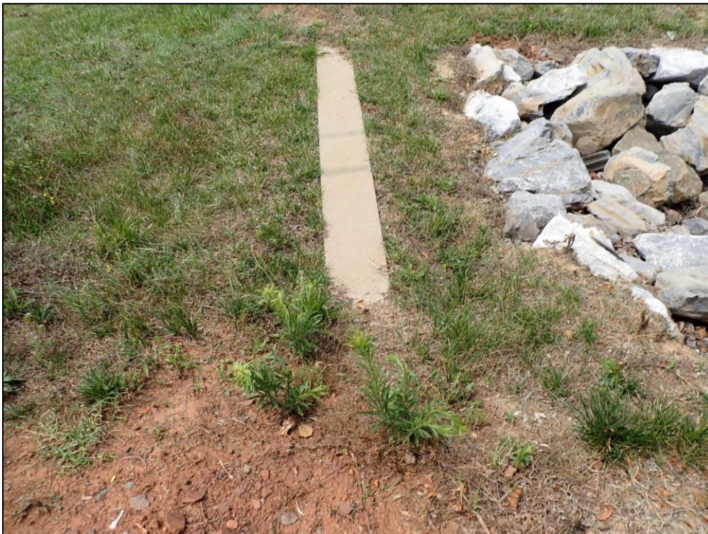
5049: Overall view of the Level Spreader. Erosion observed on the adjacent slope (Routine Maintenance Needed).
