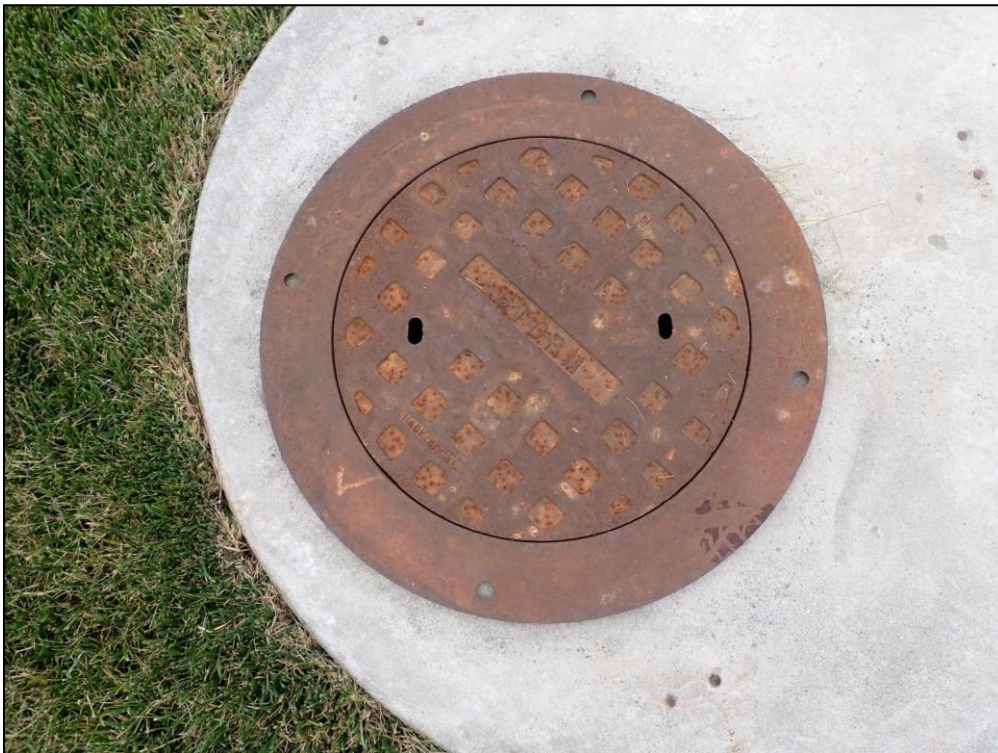
4556: Close-up of Manhole 2. Damage to the access hatch and/or ladder; the collar is not bolted down (Immediate Repair Needed).
