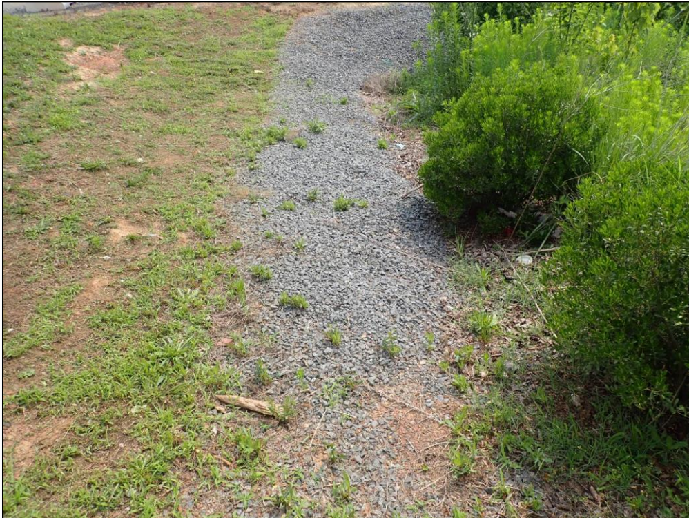
4995: Overall view of the Gravel Diaphragm. Buildup of sediment and vegetation (Routine Maintenance Needed).
