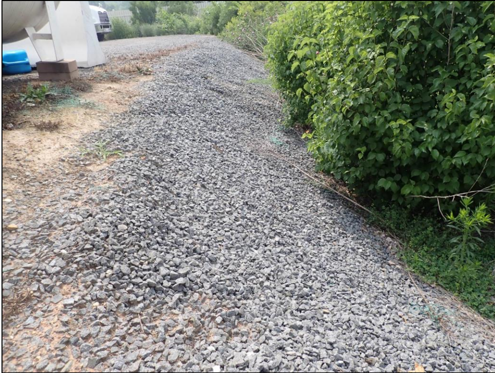
4996: Overall view of the Gravel Diaphragm. Evidence of erosion or bare spots (Routine Maintenance Needed).
