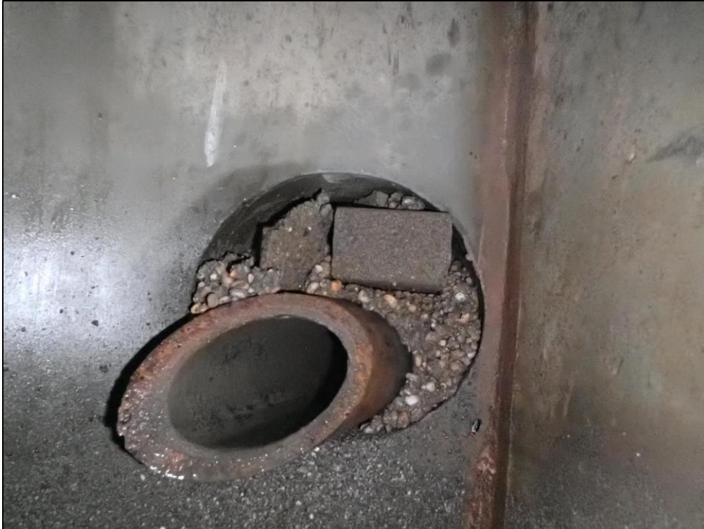
4540: Inside Control Structure 3, looking upstream toward the Cartridge Bay. Damage to outlet pipe or structure, pipe connections are not sealed (Routine Maintenance Needed).
