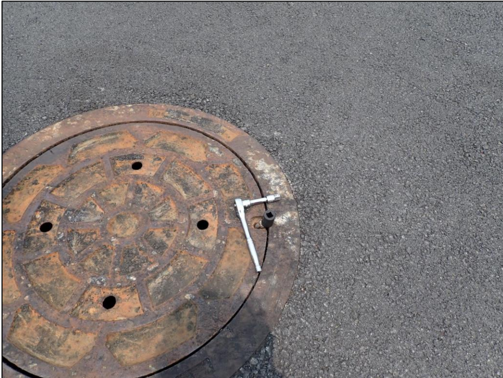
5103: Close-up of Manhole 7. Inadequate access to complete a thorough inspection, bent bolt (Routine Maintenance Needed).
