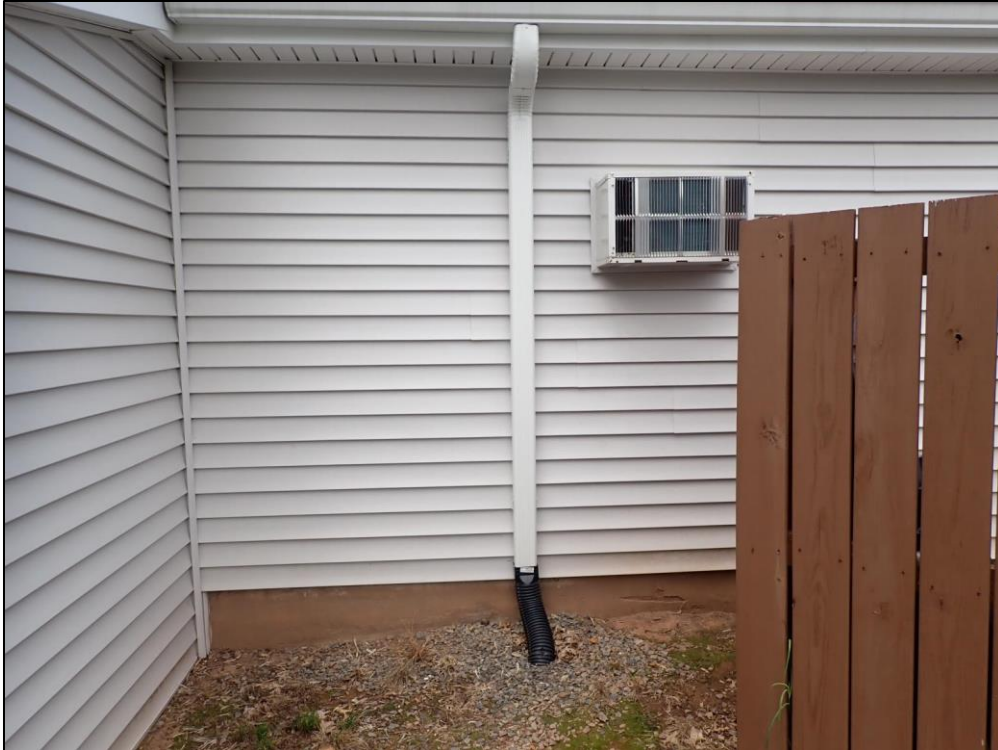
4760: Overall view of Downspout 2, piped underground toward the trench.
