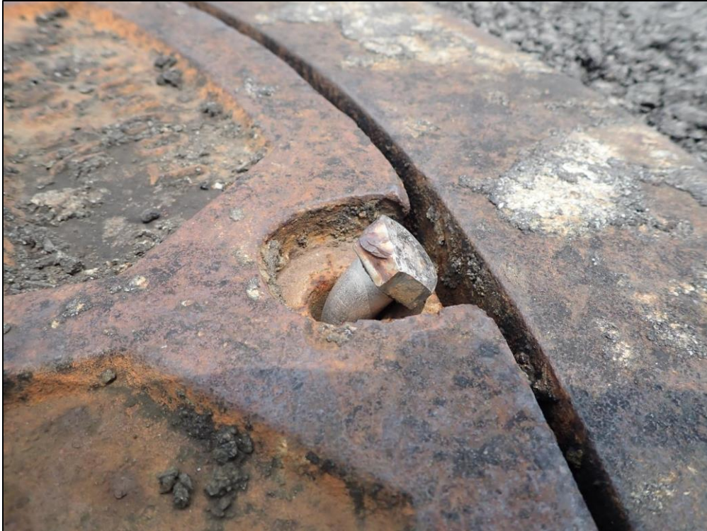
5102: Close-up of Manhole 7. Inadequate access to complete a thorough inspection, bent bolt (Routine Maintenance Needed).
