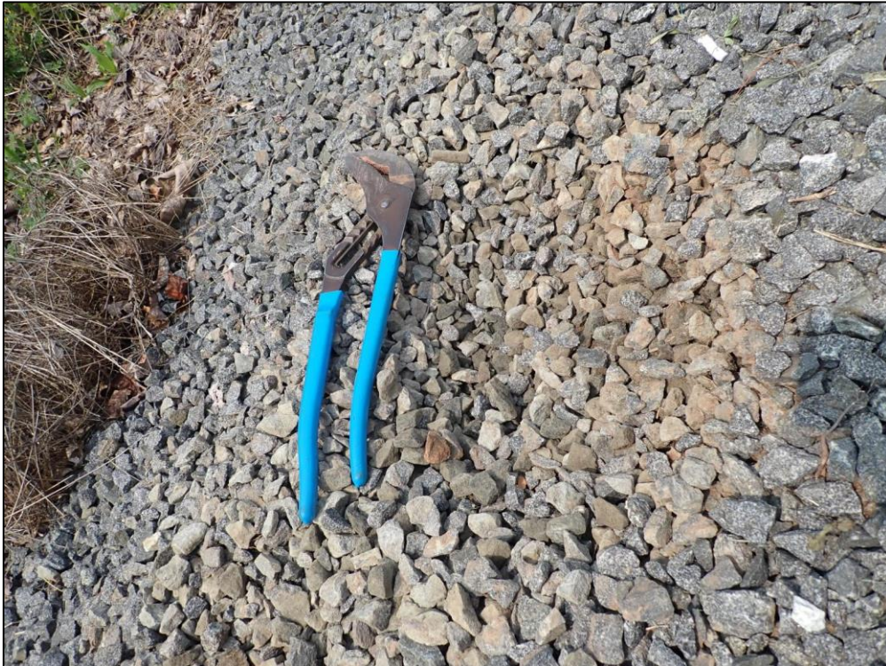
4997: Close-up of the Gravel Diaphragm, showing the gravel detail. Buildup of sediment and vegetation (Routine Maintenance Needed).
