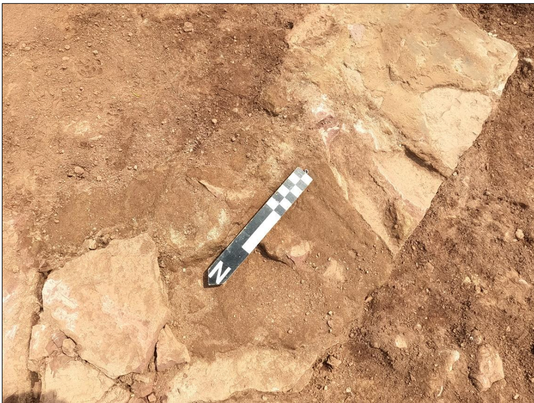
Photo 7: Detail of Mortar in Tower Foundation.
