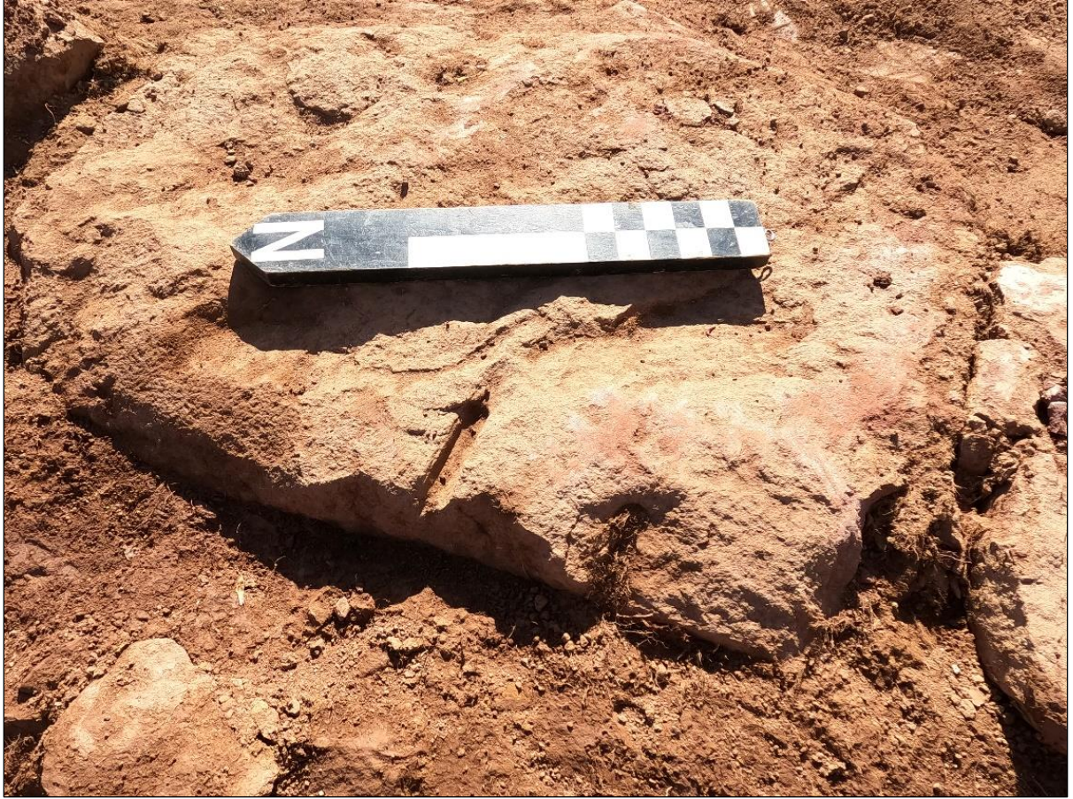
Photo 8: Blasting Hole In Stone Comprising the Tower Foundation Illustrating Pre-Construction Stone Processing Technique.
