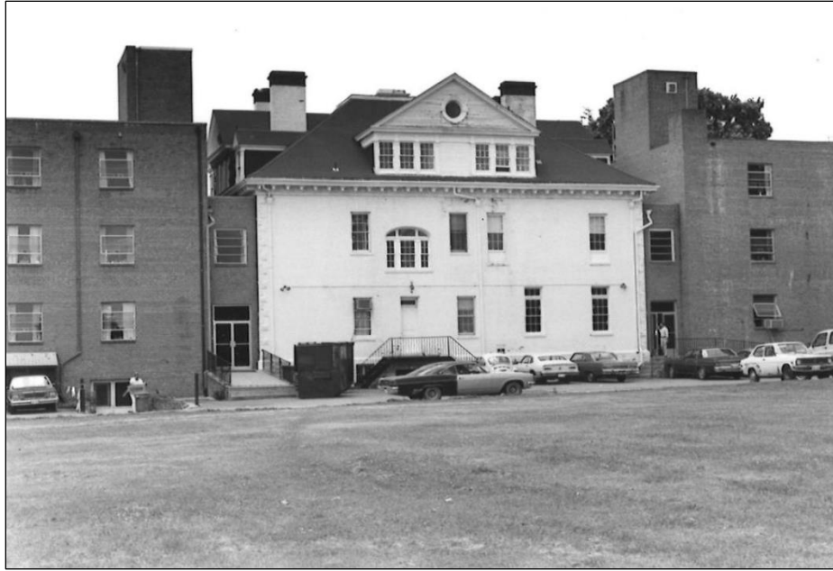
Figure 11: Rear of Annaburg, 1979 (Jones 1980). Photo shows Annaburg painted white with now-demolished wing additions.
