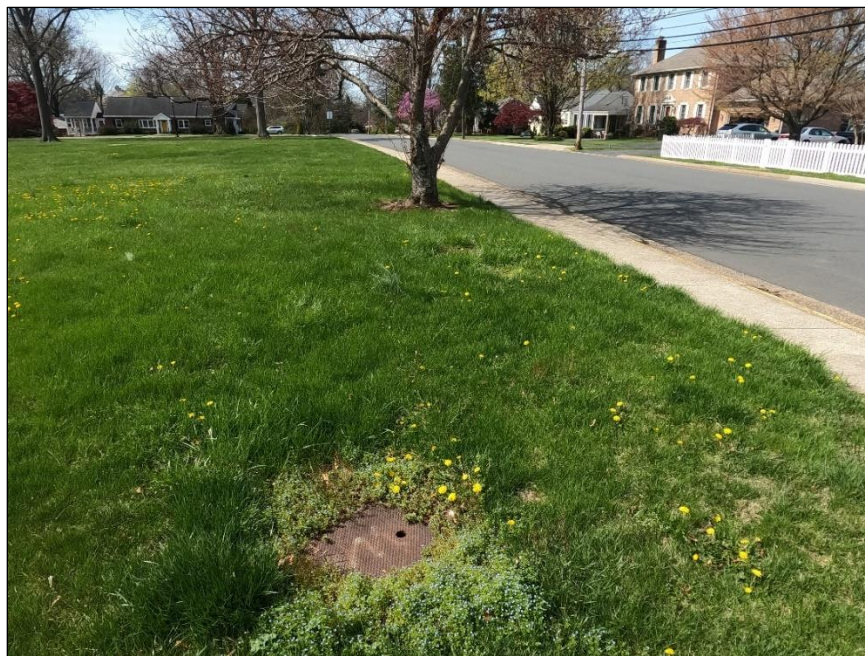
Photo 5: Sewer Cap in Northern Corner of Project Area, Facing Southwest.
