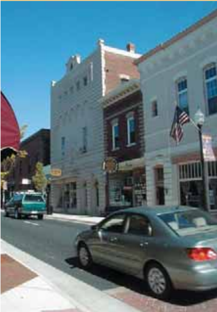
Create convenient access to upper floors with high quality residential or office uses below
