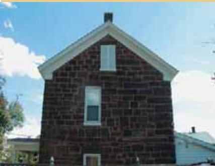
Example of a house built with sandstone; a locally quarried material used in building many of the City’s older structures.
