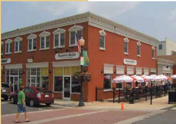
Existing 'Entertainment Zone' adjacent to the Norfolk Southern Railroad
