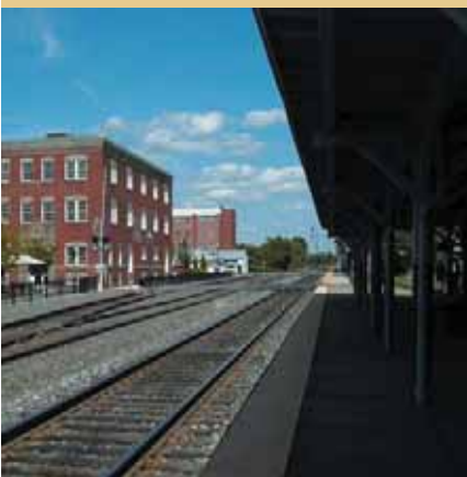
VRE/AMTRAK Train Station
