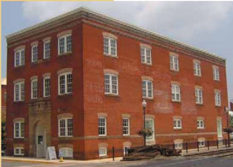
Hopkins Candy Factory restoration for city activities
