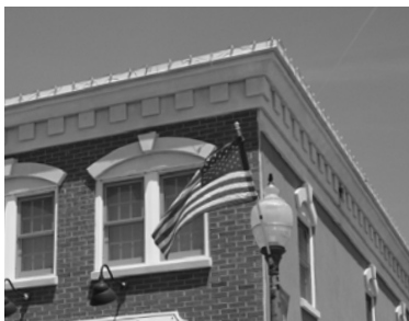
CORNICES & PARAPETS Page 130
