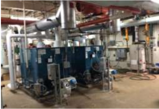
Terminal Units/Convertors: All in good shape and will last until 2029
