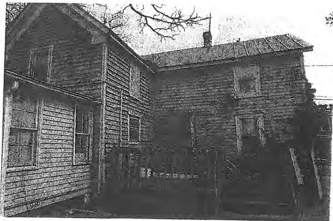
Photo #19– Deteriorated Rear Deck and Improper Foundation Support for Addition
