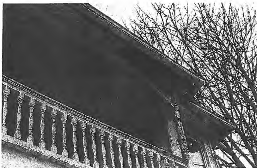
Photo #3B – Deteriorated Porch Roof
