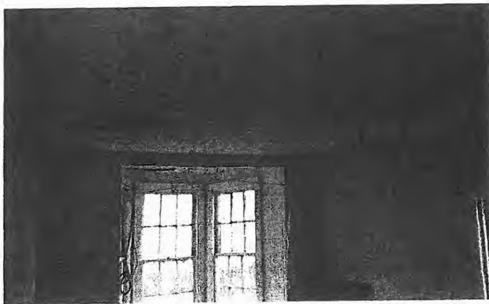
Photo #5 – Water Damage at Ceiling and Cracks in Wall Plaster
