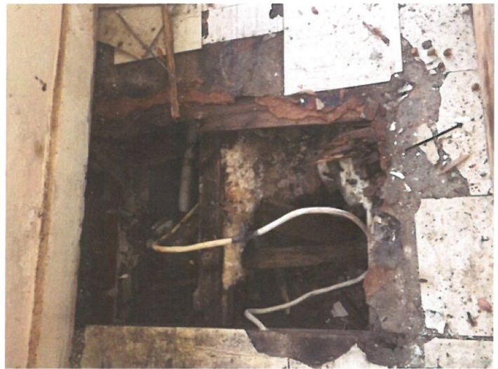
Enclosed Porch Addition Sloping and rotten support under the floor
