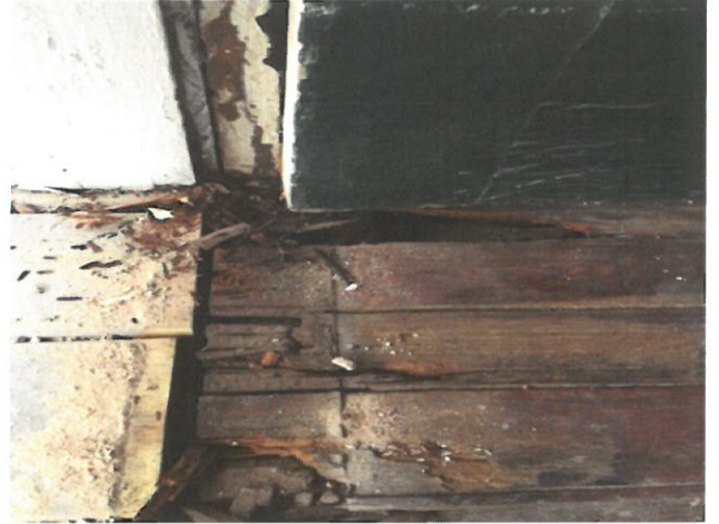
Front Door (transoms taped, floor rot, door rot)
