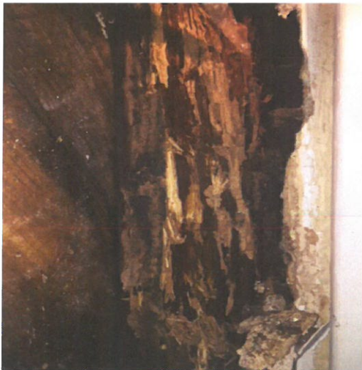
Windows – support beam adjacent to window water damaged and rotting – another window with wood rot
