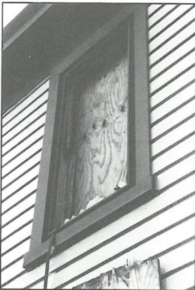
This window has been blocked in and the loosely applied plywood allows water infiltration.
