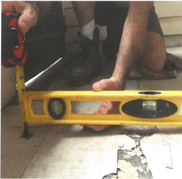
Enclosed Porch Addition Sloping and rotten support under the floor
