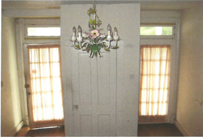
Front Door (transoms taped, floor rot, door rot)
