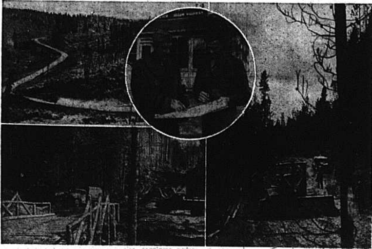
U. S. troops and supplies are now rolling into Alaska over the Alaska Highway (Alcan), which was finished months ahead of schedule. The 1,600-mile road ends at Fairbanks. Photos show (right), a bulldozer knocking a trail through virgin forest; lower left, a "carry-all" puts the finishing touches to a section of the highway as trucks bring up gravel for surfacing; upper left, scenic view of the Alcan as it winds through the Yukon. Circle: Brig. Gen. William Hoge and Maj. E. J. Stann, executive officer, discuss route at Whitehorse.
