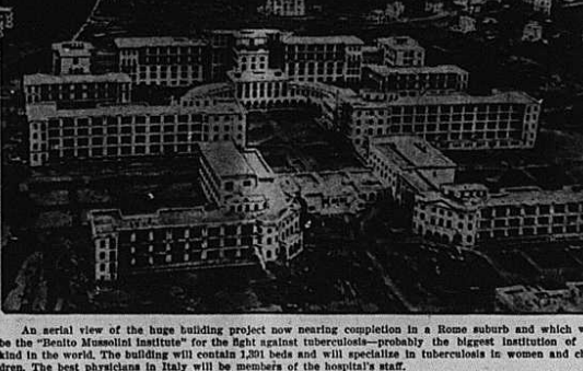
An aerial view of the huge building project now nearing completion in a Rome suburb and which will be the "Benito Mussolini Institute" for the fight against tuberculosis...
