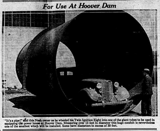
"It's a pipe" said this Nash owner as he wheeled his Twin Ignition Light into one of the plant tubes to be used in equipping the power house at Hoover Dam. Measuring over 13 feet in diameter this huge conduit is nevertheless one of the smallest which will be installed. Some have diameters in excess of 30 feet.
