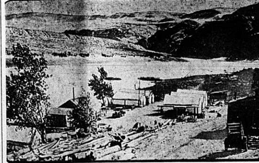
Here is the first construction camp at the site of the Grand Coulee dam on the Columbia river, where drillers and surveyors engaged on the preliminary steps to the project are housed. A year from now several thousand workmen are expected to be quartered here as the construction work goes forward. The project will cost $23,000,000.
