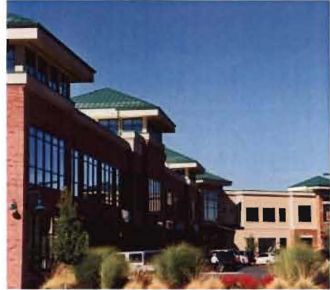
Required: Varied roof forms and depth help to reduce perceived building scale. False roof forms shall have depth behind the façade of the building no less than 25 % of the depth of the building footprint.
