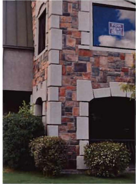
Required: Use a variety of materials and alterations in the façade to clarify entries and reduce the perceived building scale.
