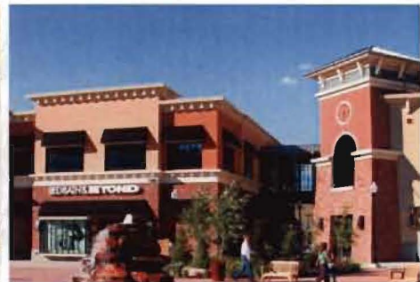
Example: Varied roof forms, heights, design details, and materials can be used to clarify entrances and reduce perceived building scale.
