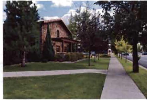
Example: Integrating a variety of forms helps reduce the mass of a building.
