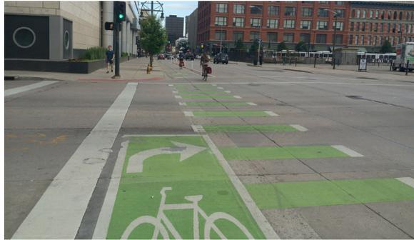
Figure 4.17 Typical two-stage turn queue box
