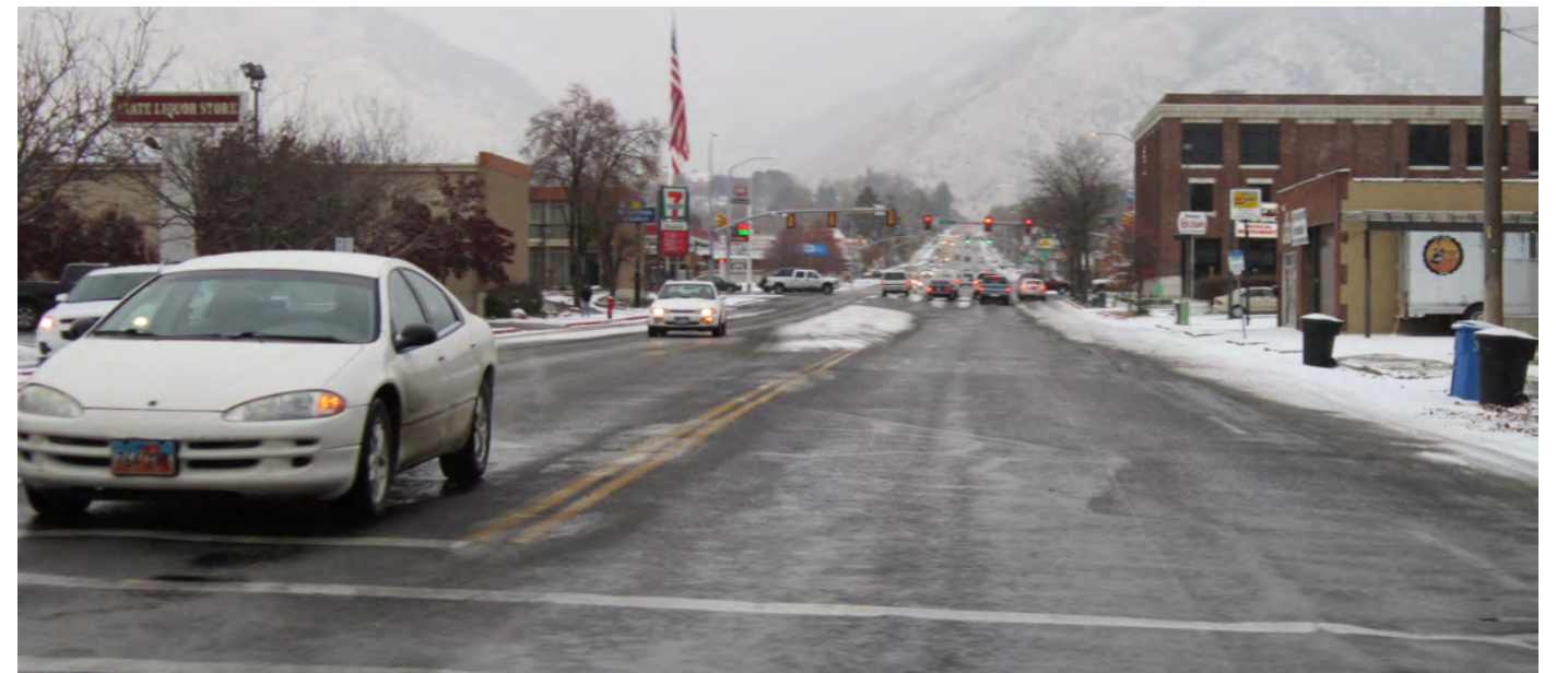
The Fourth North corridor, is generally characterized by 2 11-foot travel lanes in each directions with a center turn lane. Sidewalks are 4 to 5 feet in width, with a narrow park strip of 3 to 4 feet. View from 100 West, looking east.
