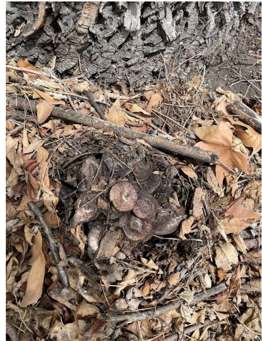
Figure 5 Armillaria at base of tree
