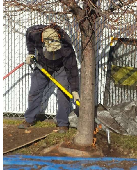
Figure 6 Root excavation with air tool
