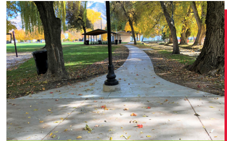
Central Park Sidewalk Project
