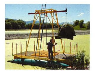
The images above show the service barge being used to pull out (left) a Bio-Dome and deliver it to the shore (right) from the Wellsville UT installation as part of an upgrade to the latest and most efficient air distribution hose.
