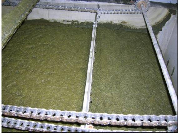
Figure 12. Clari-DAF System Sludge Blanket and Skimmer.
