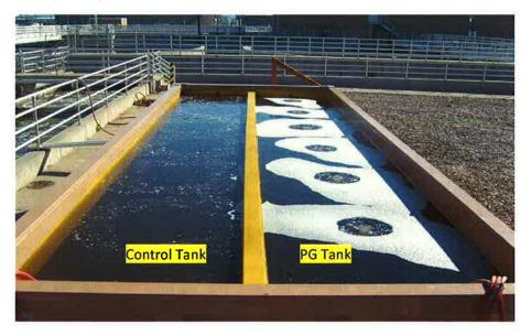
Figure 3: Reactor tanks in operation since mid-October, 2010. Effluent holes are visible at the far end. Wastewater Compliance Systems, Inc Proprietary Information ©2011
