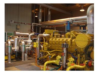
800 kW Caterpillar Digester Gas-Fueled Cogeneration System, Sunnyvale, CA WWTP
