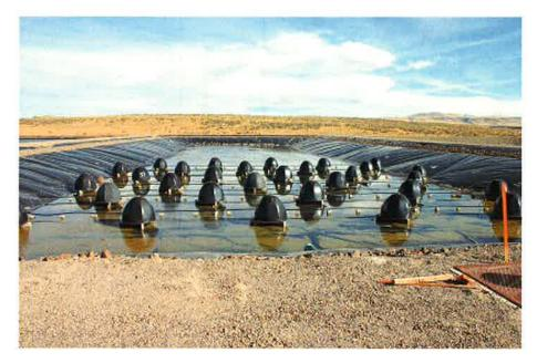
Figure 23 - Installation of Poo-Gloo Units in Cell 2 in Jackpot, Nevada
