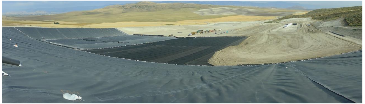
One 10-acre cell of the North Valley Landfill in the process of being lined in 2017
