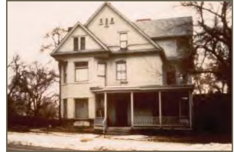
Avenues home before rehabilitation, Salt Lake City
