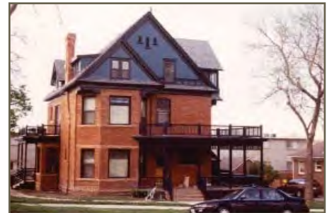
Avenues home after rehabilitation, Salt Lake City
