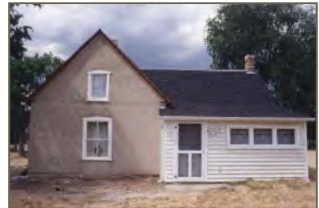
Spring City home after rehabilitation
