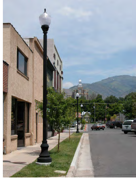
This building façade with its extensive use of stucco and lack of historic design elements are not in character with the traditional building design found in downtown Logan
