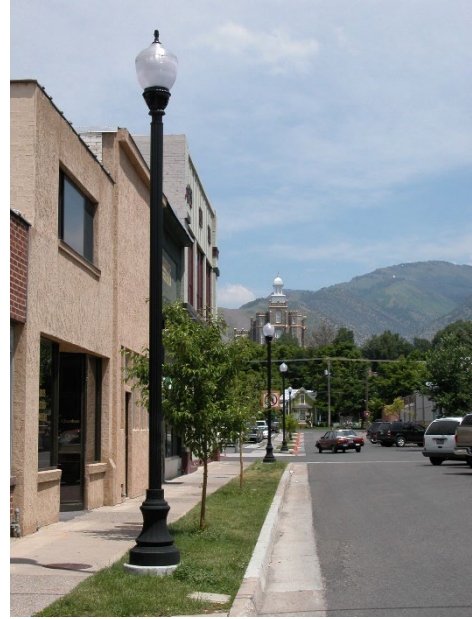
This building façade with its extensive use of stucco and lack of historic design elements are not in character with the traditional building design found in downtown Logan
