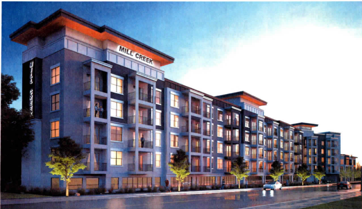
Figure 1 shows Millcreek Phase 2 along 100 South.
