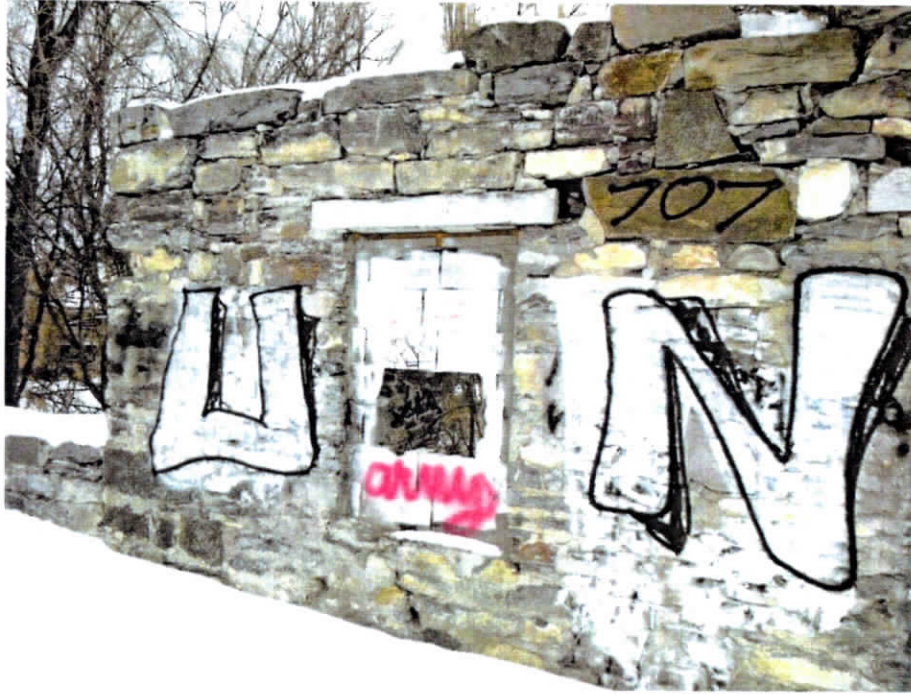
Photo 1 CMU masonry infill
