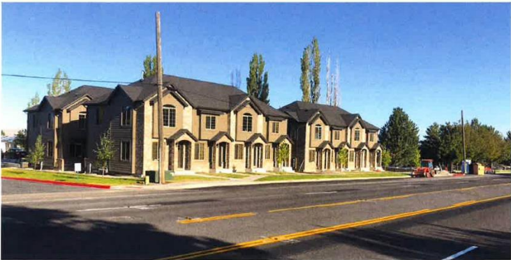
PREVIOUS BUILD AT 1325 NORTH 800 EAST, LOGAN
