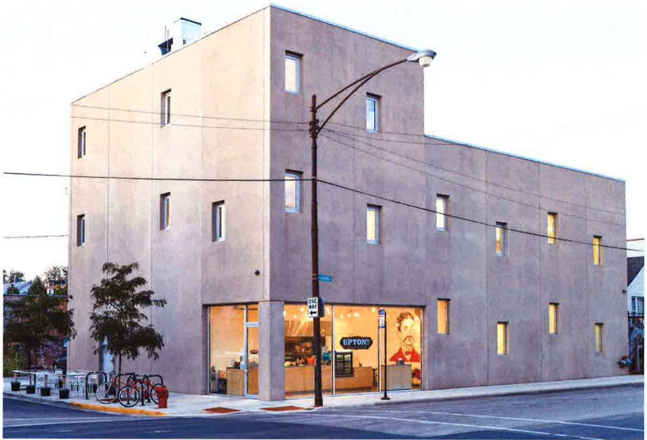
Decorative concrete – aesthetic finish with no structural function
