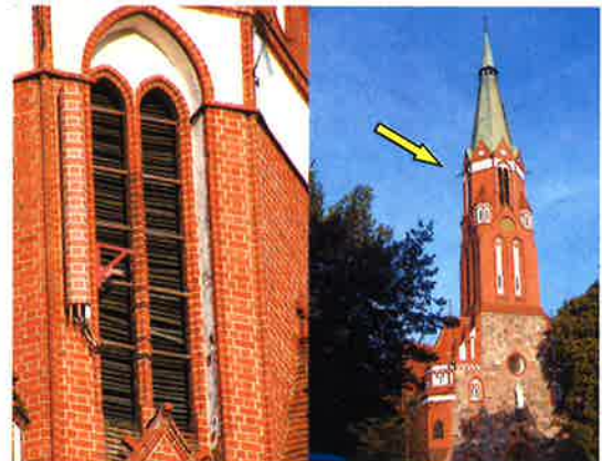
Example of a Stealth Design by placing equipment on Existing Buildings
