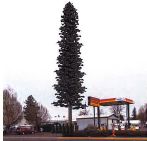
Example of Using Stealth Design with a Tower constructed to simulate an Evergreen Tree with Vegetation
