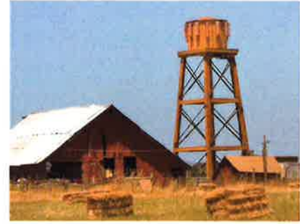
Example of a Stealth Design by placing equipment on existing Agricultural Structures
