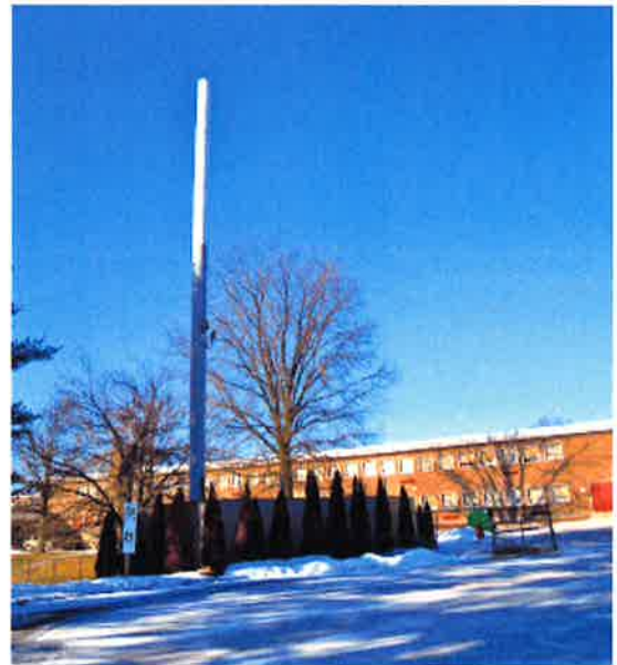
Stealth Design on Existing Buildings with Monopole (antennas inside pole)
