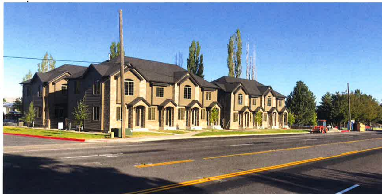
PREVIOUS BUILD AT 1325 NORTH 800 EAST, LOGAN
