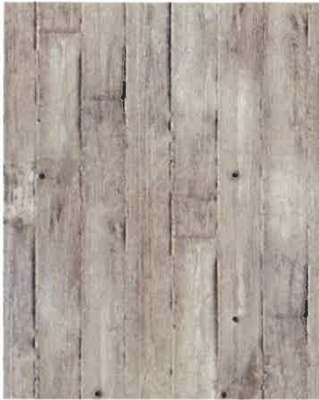
BOARD FORMED CONCRETE SMOOTH HORIZONTAL
