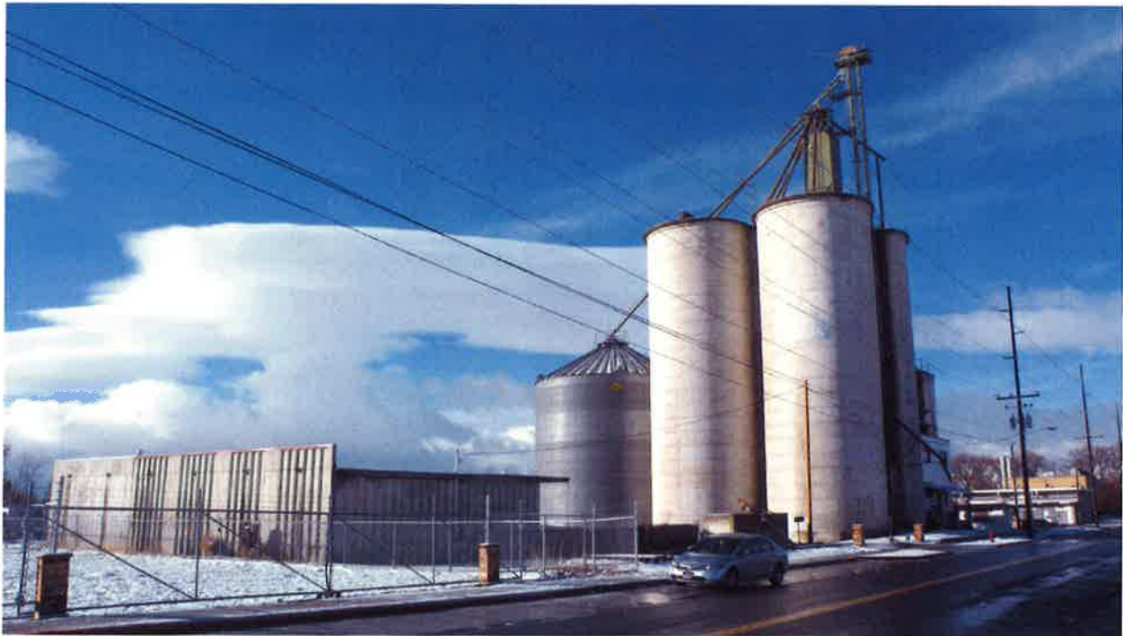
The Barn existing building – East and North elevation, adjacent silos
