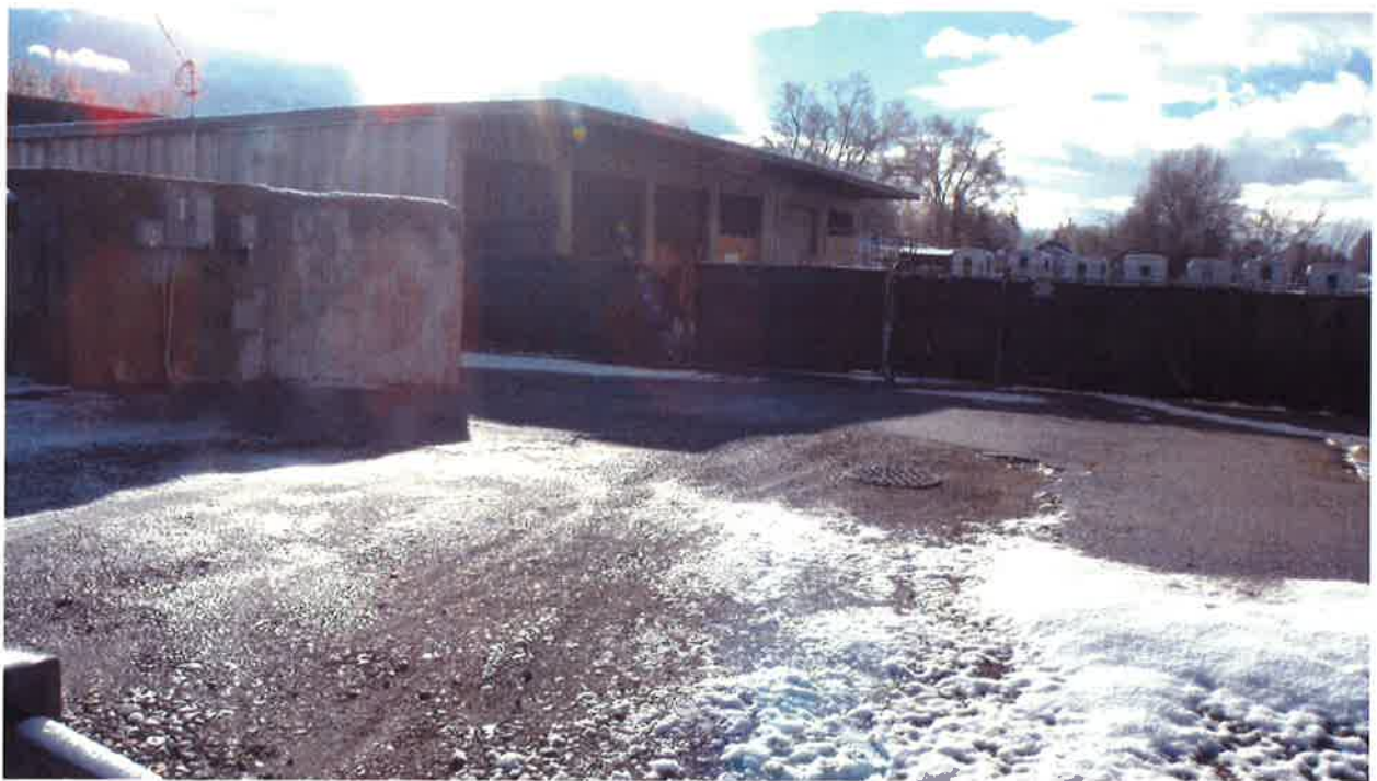
The Barn existing building – West elevation
