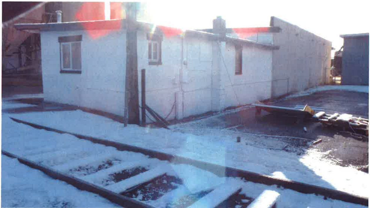
The Homestead existing building – North and West elevation
