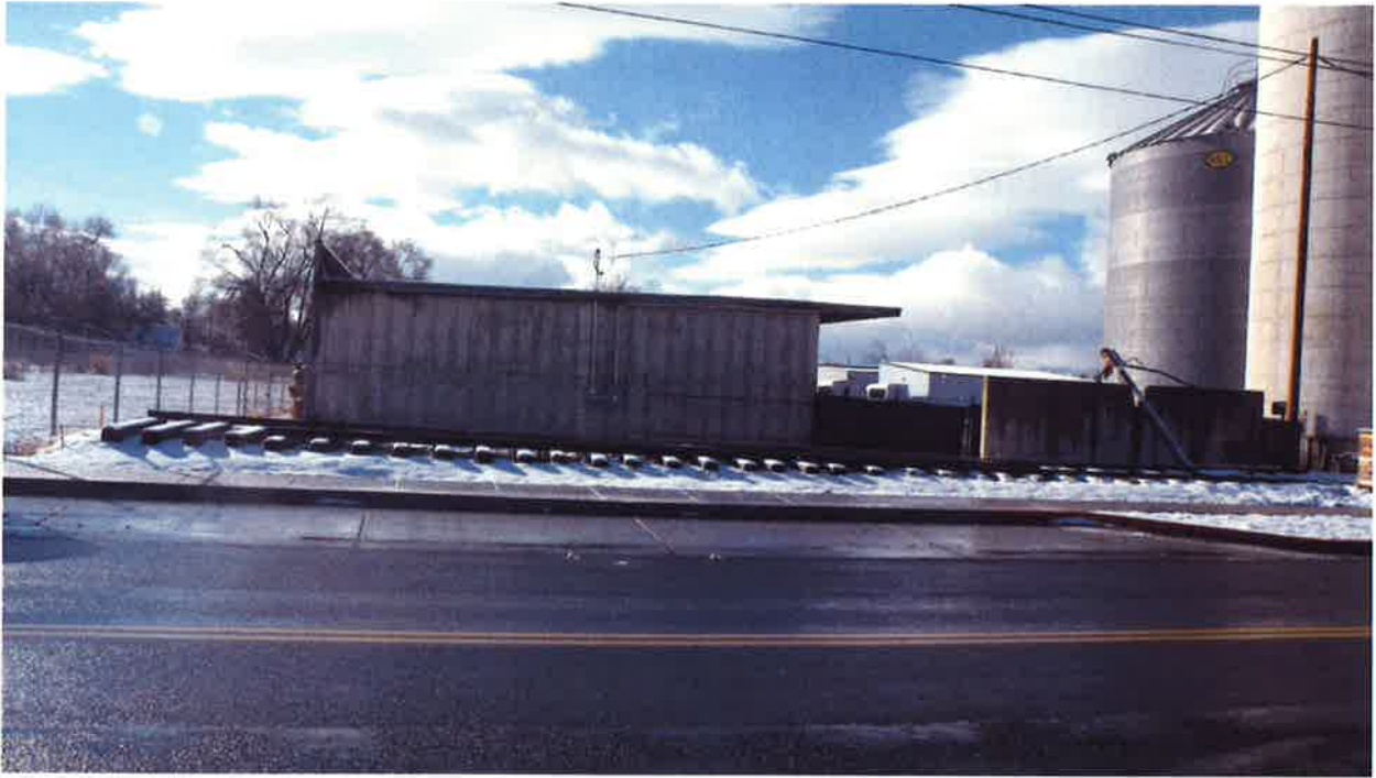
The Barn existing building – North elevation
