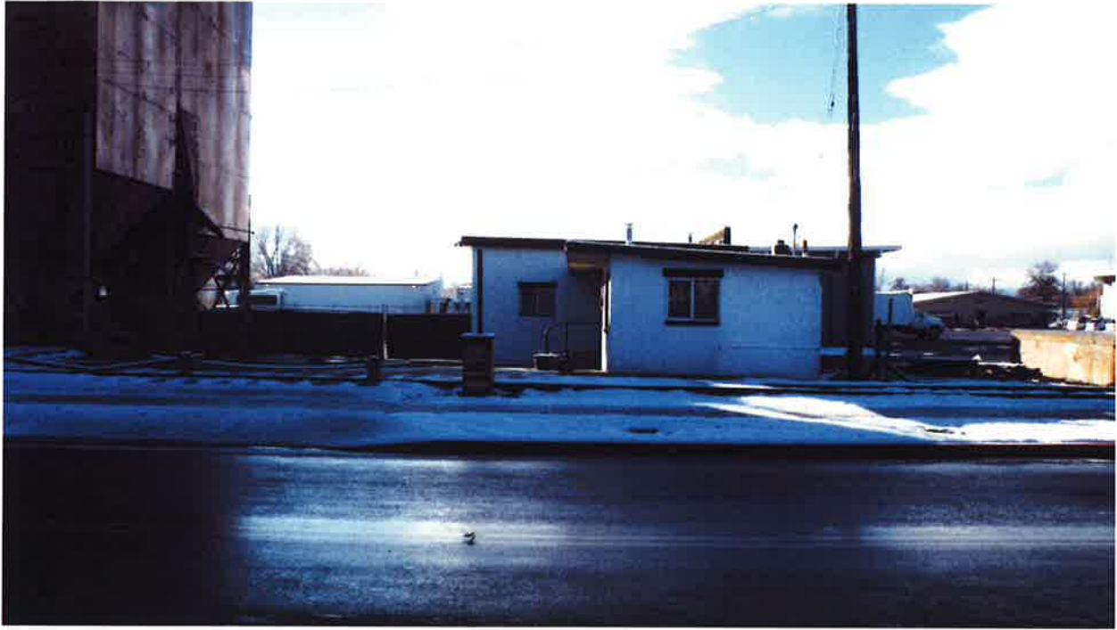
The Homestead existing building –North elevation
