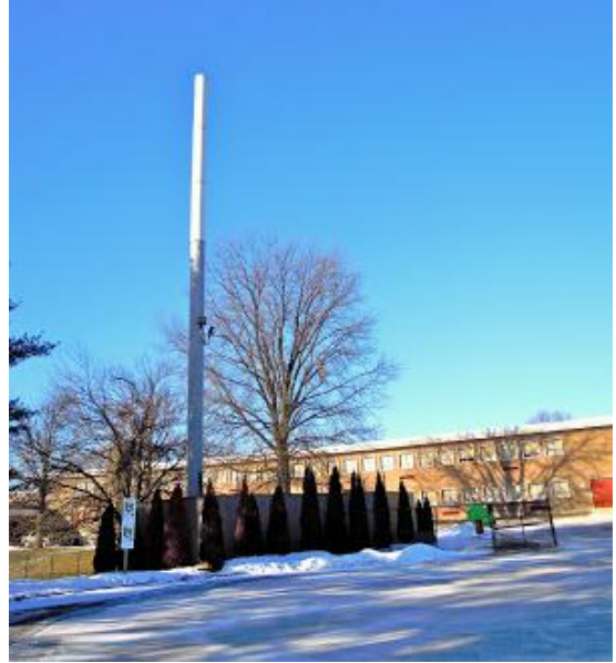
Stealth Design with Monopole (antennas inside pole)
