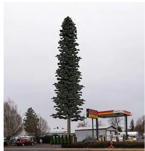
Example of Stealth Design with a Tower constructed to simulate an Evergreen Tree
