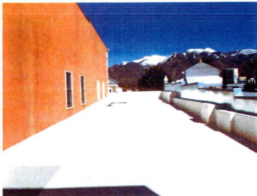
Figure S-8 Building 41 Roof Facing East.
