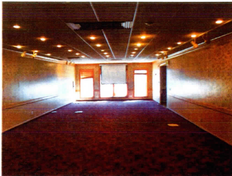
Figure S-44 Building 67 2nd Floor.
