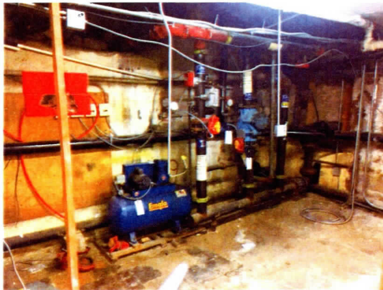
Figure S-23 Building 59 Basement.
