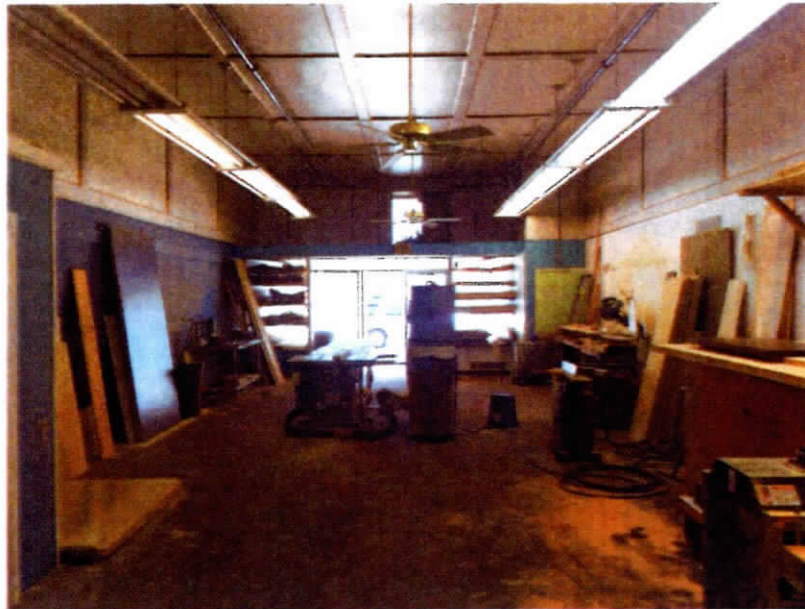
Figure S-41 Building 67 Main Floor Facing East.
