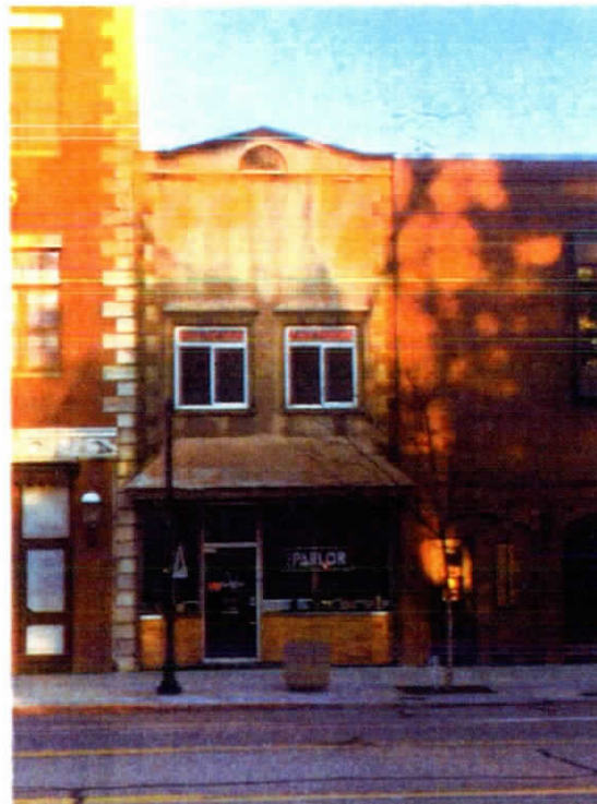
Figure S-17 East Elevation of Building 47.
