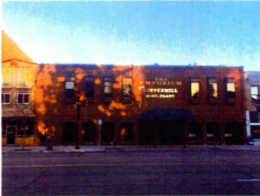
Figure S-22 East Elevation of Building 59
