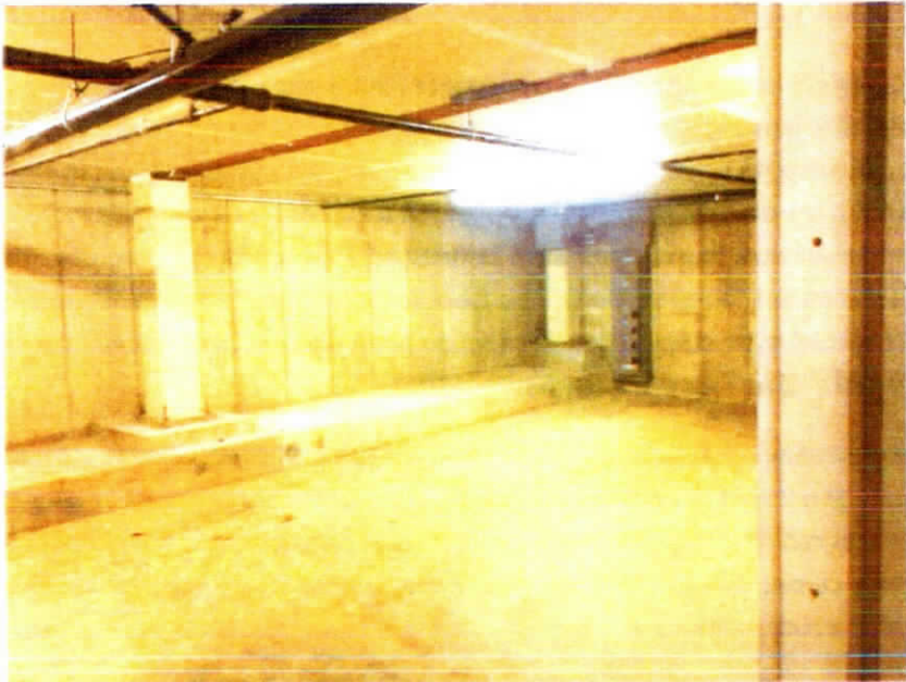
Figure S-10 Building 45 Basement
