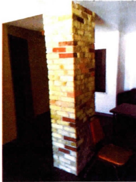
Figure S-26 Building 59 Basement Masonry Column.
