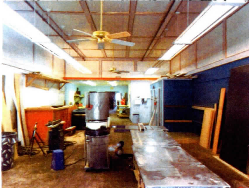
Figure S-42 Building 67 Main Floor Facing West.
