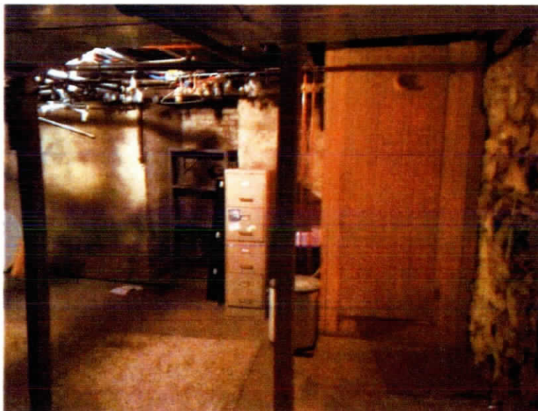
Figure S-40 Building 67 Basement Facing North.
