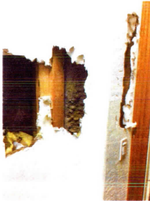
Figure S-43 Building 67 West End of 61 ft Concrete Wall.
