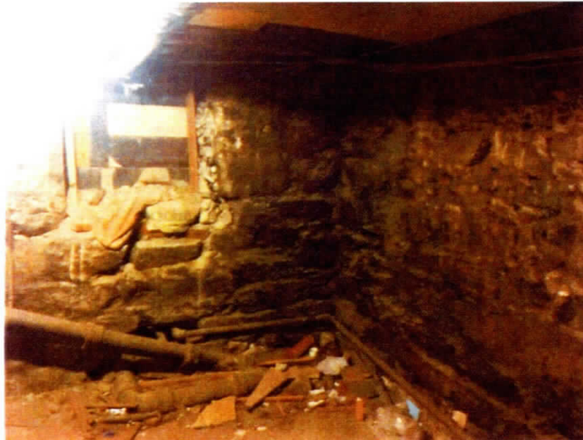
Figure S-38 Building 67 Basement Facing West.
