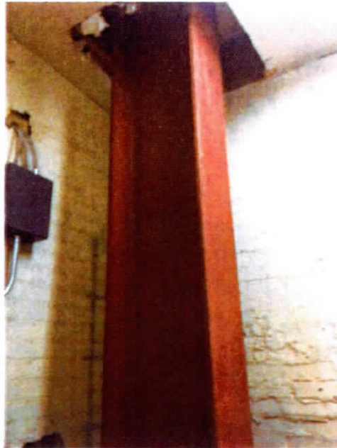
Figure S-12 Moment Frame Inside South West Wing of Building 45.
