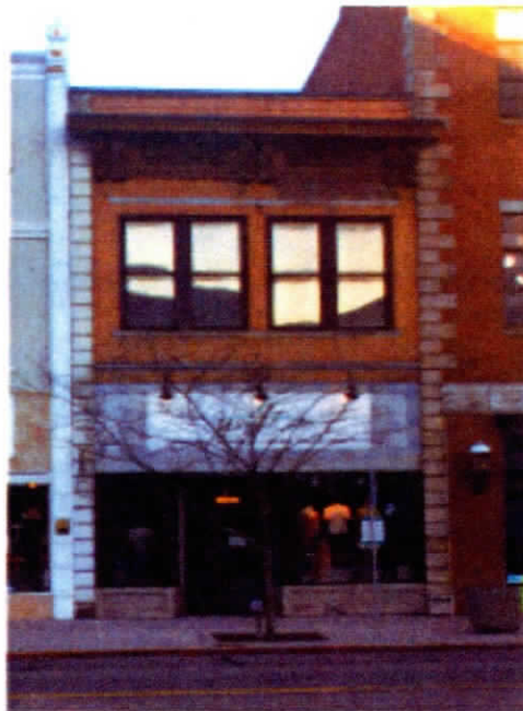
Figure S-2. East Elevation of Building 41
