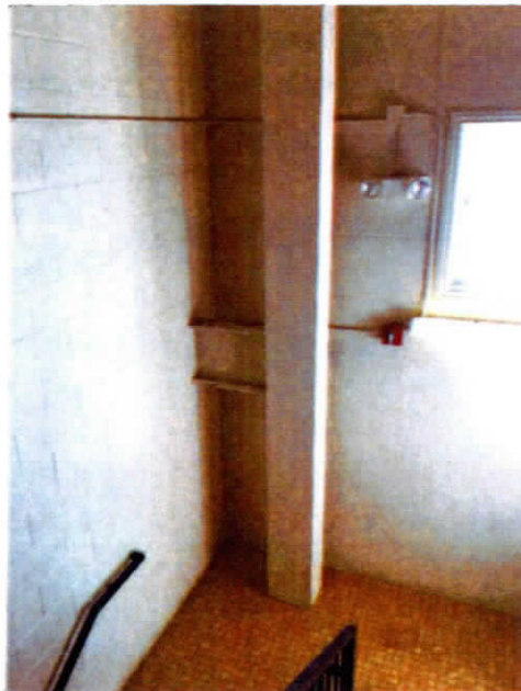
Figure S-13 Building 45 Stair.
