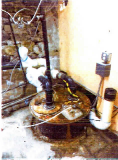
Figure S-24 Building 59 Sump Well in Southeast Corner.
