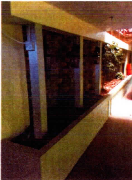
Figure S-25 Building 59 Basement Rock Bearing Wall.
