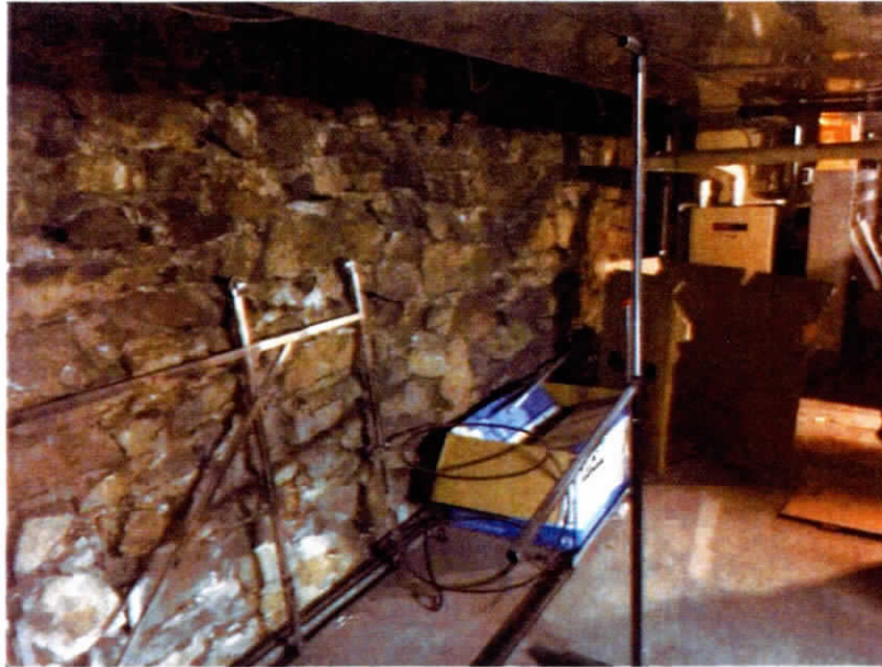
Figure S-18 Building 47 Basement.
