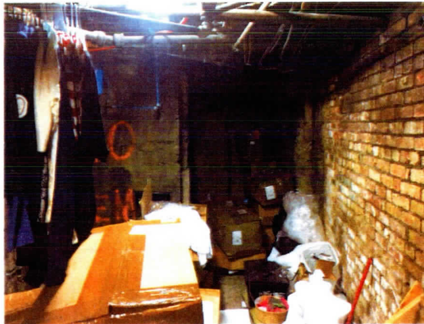
Figure S-4 Building 41 Basement Looking West.
