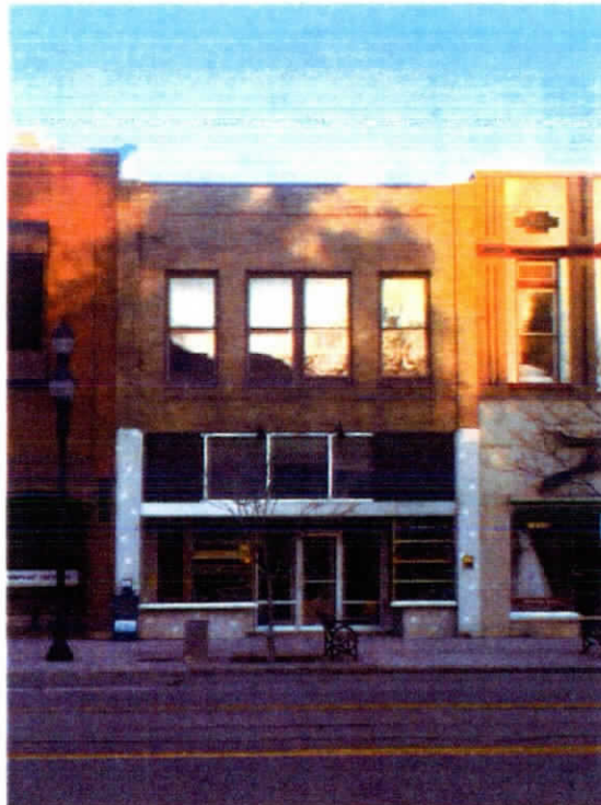
Figure S-36 East Elevation of Building 67.
