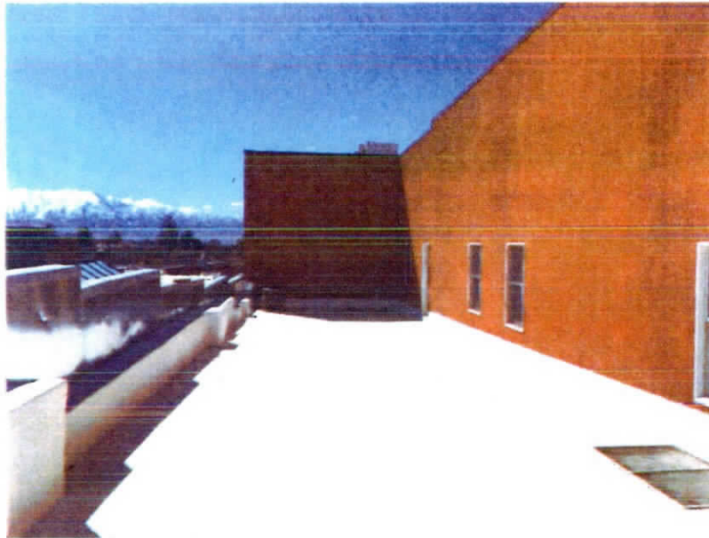
Figure S-7 Building 41 Roof Facing West.
