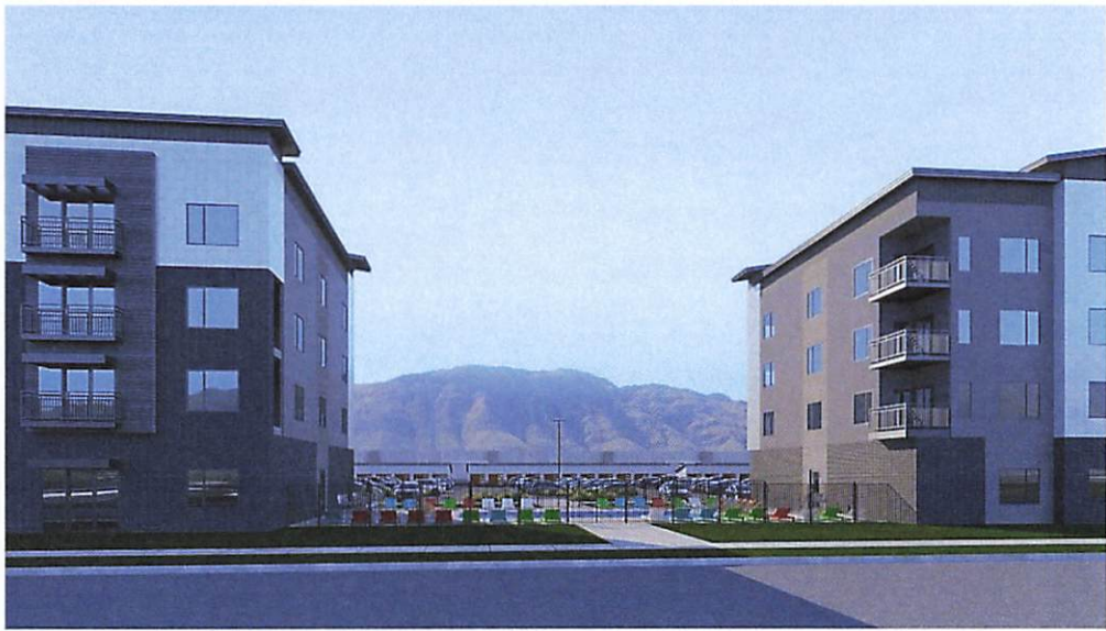
View West from N 200 E Road
