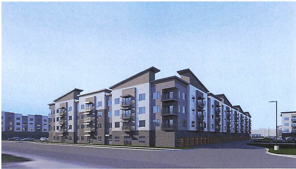
View Northwest from E 1250 N Road
