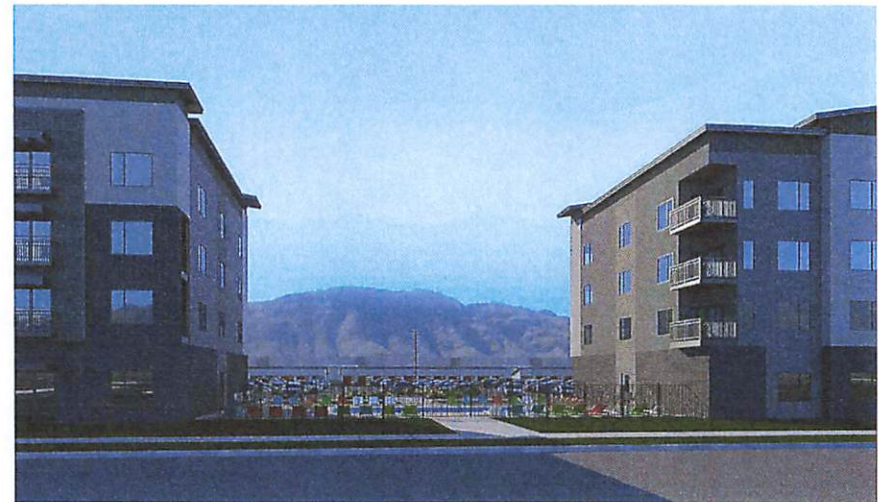
View West from N 200 E Road
