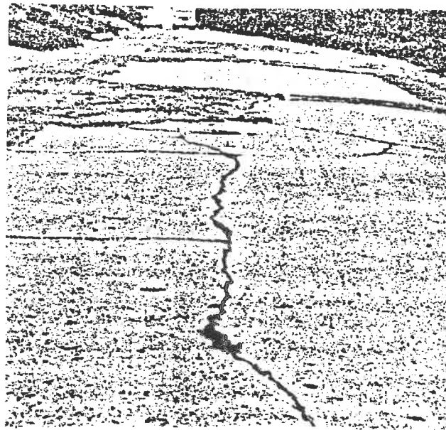
Figure 13. LONGITUDINAL CRACK
