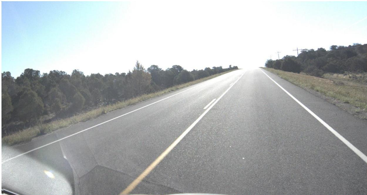
**CR 318 from Called Brazo to Jaques Drive (GISID 1551, PCI = 95)** – Rated as Excellent, this pavement displays little to no surface distresses. The ride is smooth, and the surface and the base are intact. Excellent roads should be periodically assessed for crack development that would trigger routine maintenance activities.
