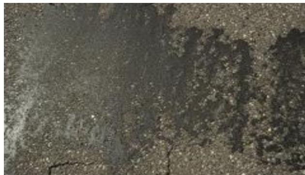
**Edge Cracking** – Running parallel to the road and usually within 1 to 2 feet of the outer edge of the pavement, this distress is caused by traffic loading and weakened base conditions resulting from poor drainage. It is measured in linear feet.
