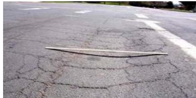
**Longitudinal & Transverse Cracking** – Quantified by their length and width. These cracks can be the result of pavement shrinkage due to natural daily and seasonal temperature cycles, construction issues, or other factors.
