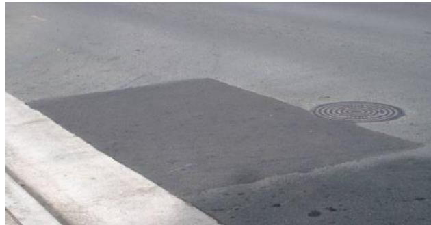
**Raveling** – This is the loss of coarse aggregate on the pavement surface and is measured by the severity and square footage affected.
