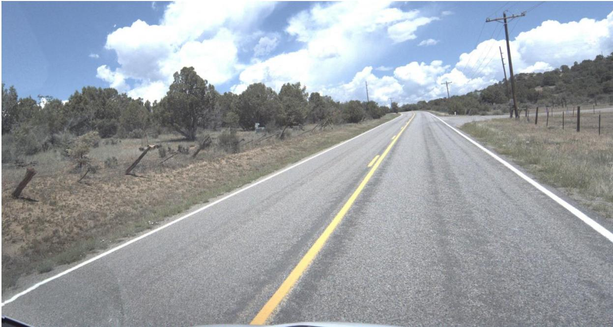
**CR 223 from Hollow Ridge Road to Private Oil and Gas Access (GISID 1615, PCI = 76)** – Rated as Very Good, this road displays minor amounts of longitudinal cracking. This street is an example of a candidate for preventative maintenance such as microsurfacing to extend the life of the roadway.
