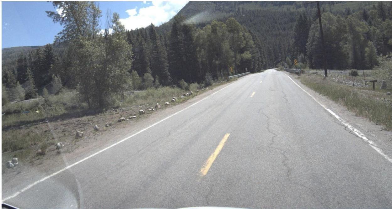
**CR 501 from Mushroom Lane to Tucker Lane (GISID 1860, PCI = 47)** – On this street, the primary cause of deterioration is the edge cracking and longitudinal cracking that is present along the majority of the segment.
