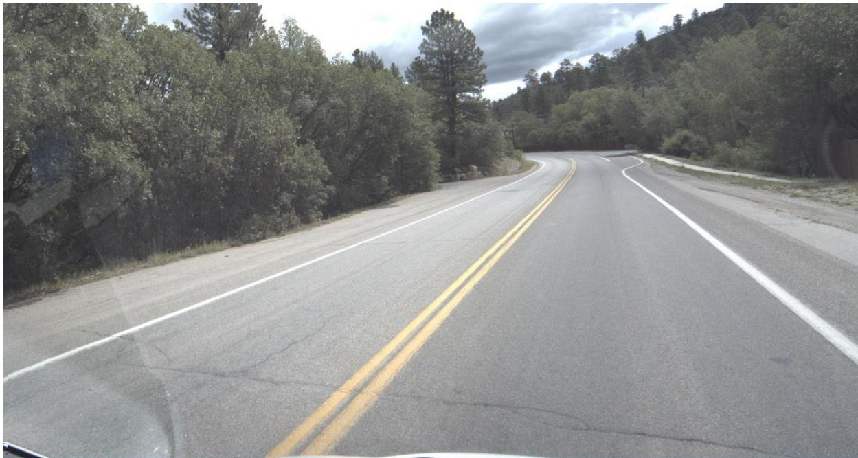
**CR 240 from Timberline Drive to Elkridge Lane (GISID 1870, PCI = 67)** – Rated as Good, the primary cause of deterioration is the transverse cracking. The pavement surface could be restored further with additional spot patching to fully waterproof the pavement.
