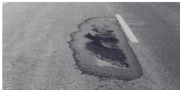
**Weathering** – This is the wearing away of asphalt binder and fine aggregate matrix, which is quantified by severity and square footage.
