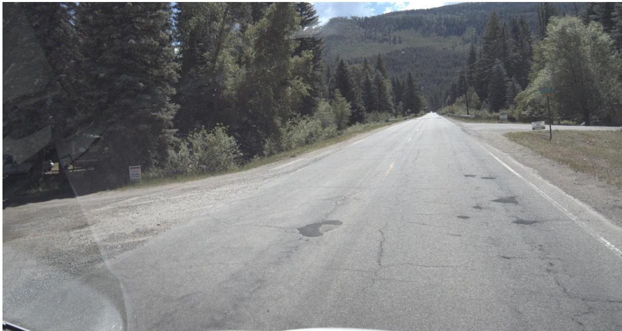
**CR 501 from Hummingbird Way to Vallecito Creek Road (GISID 1864, PCI = 37)** – Rated as Poor, this segment still has some remaining life before it becomes a critical reconstruction need. As evident in the imagery, a fair amount of the segment is severely cracked with some potholes present that have been previously filled. If left untreated, within a short period of time, a partial to full reconstruction would be required.
