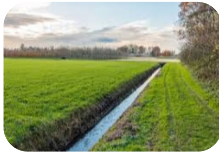
Ditch moves stormwater above ground
