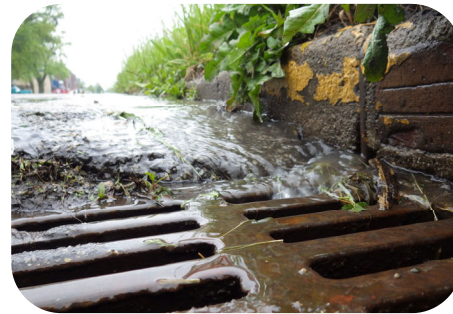
Inlet moves stormwater below ground
