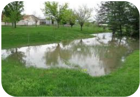
Basin captures stormwater
