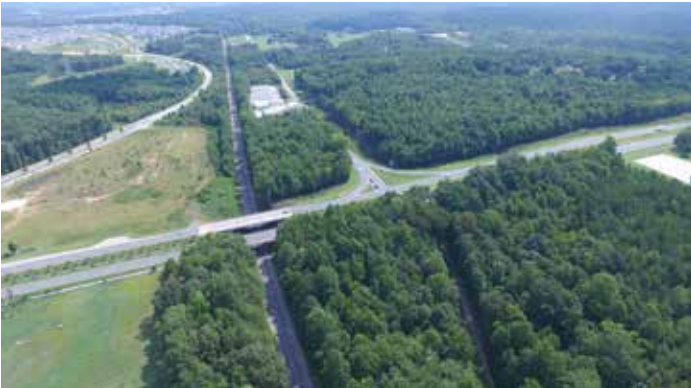
Northern area, US 521, view West of CSX Railroad and Highway 75
