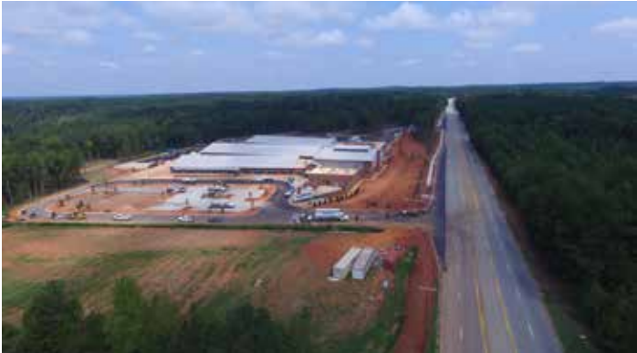
US 521, view North at Van Wyck Elementary School
