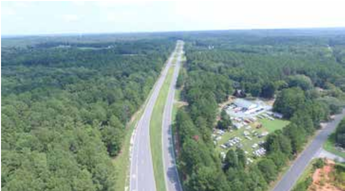
US 521 at East Rebound Road, view North
