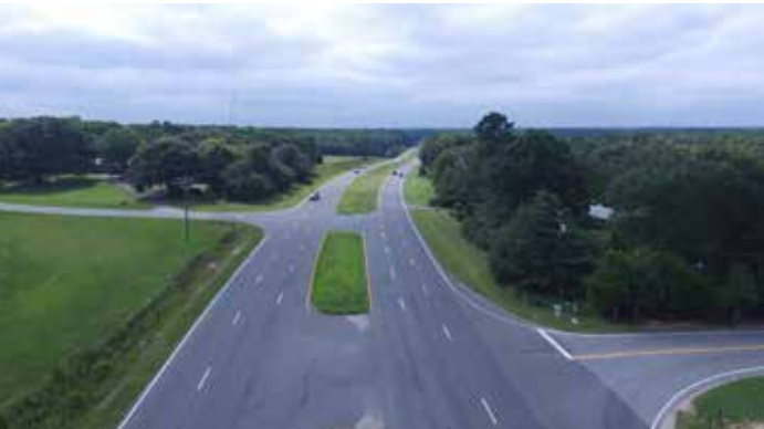
Intersection area of US 521 and Steele Hill Road and Nivens Road, view South
