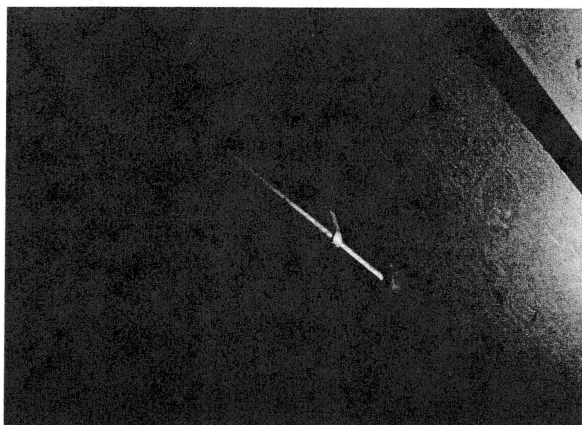
EXPOSED SPRINKLER PIPING WITH UPRIGHT HEAD
