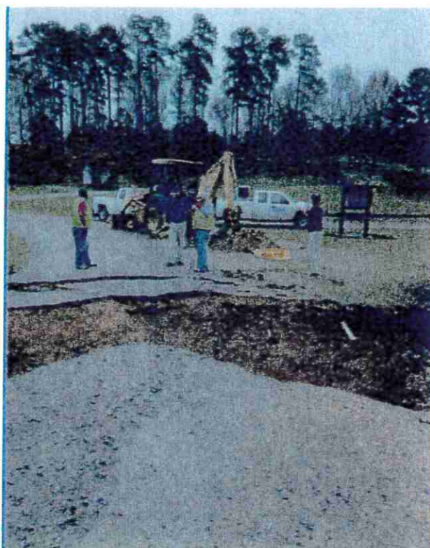
Fig. 3 -16 Fish Hatchery Road November 2015 (Hanging Rock Creek) Road failure due to extreme wash downstream from an earthen dam.
