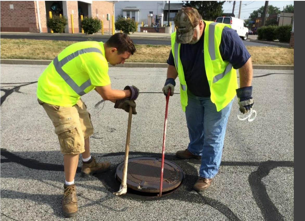
Lakewood staff opening an underground SCM for inspection.
