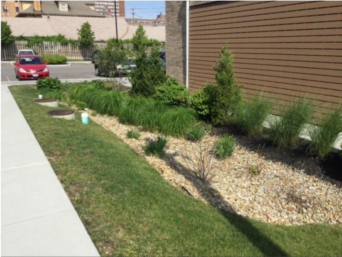
A local bioretention basin in Lakewood.
