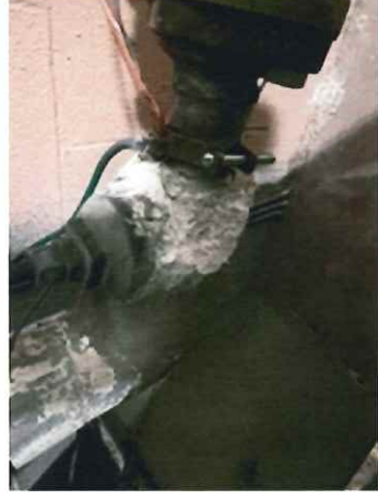
Picture 3 – Pipe w/Crumbling Insulation
