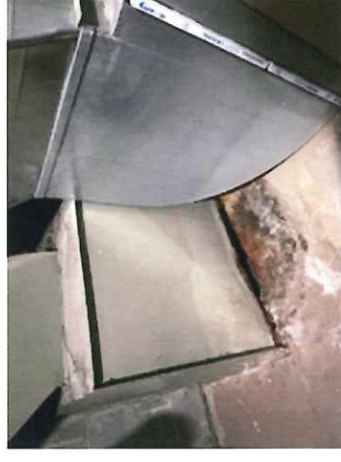
Picture 4 – Rusted Ductwork w/Opening
