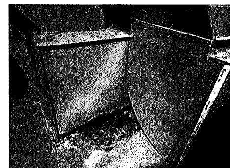
Picture 4 – Rusted Ductwork w/Opening
