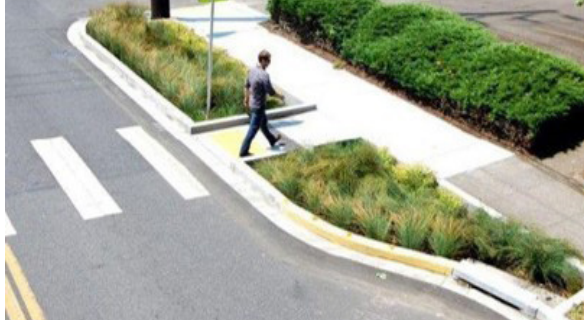
Stormwater Curb Extension
