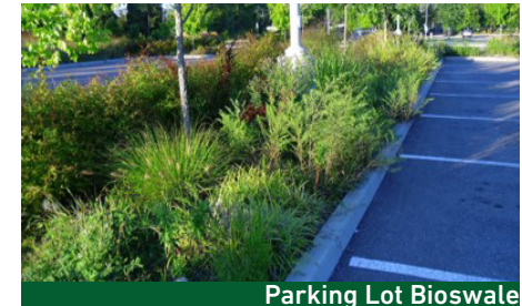
Parking Lot Bioswale
