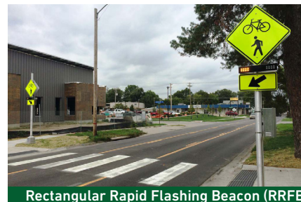
Rectangular Rapid Flashing Beacon (RRFB)
