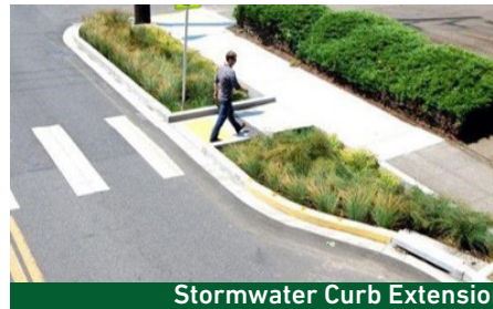
Stormwater Curb Extension
