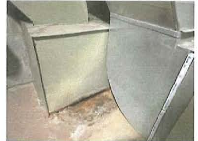
Picture 4 – Furnace Return Air Opening
