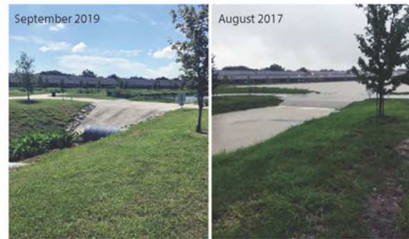
Exploration Green constructed stormwater wetland (Clear Lake, TX) on a typical day (left) and during Hurricane Harvey flooding in 2017 (right).
