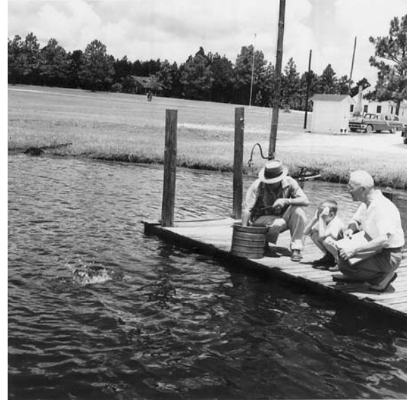
Figure A-9. The Lyman Fish Hatchery just after its opening
