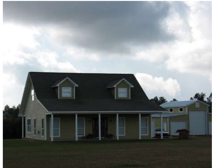
Figure A-21. The house shown below is typical of many homes in Western Harrison County.
