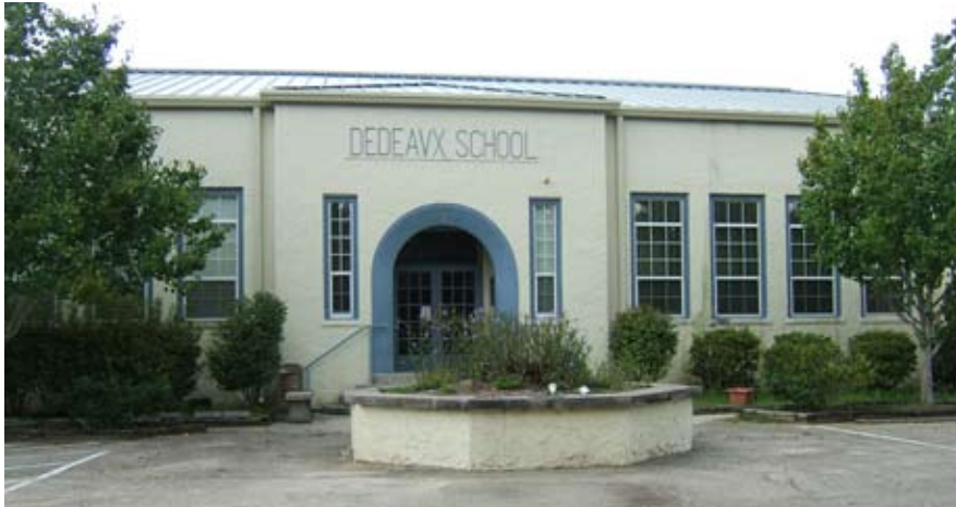
Figure A-10. The original Dedeaux School
