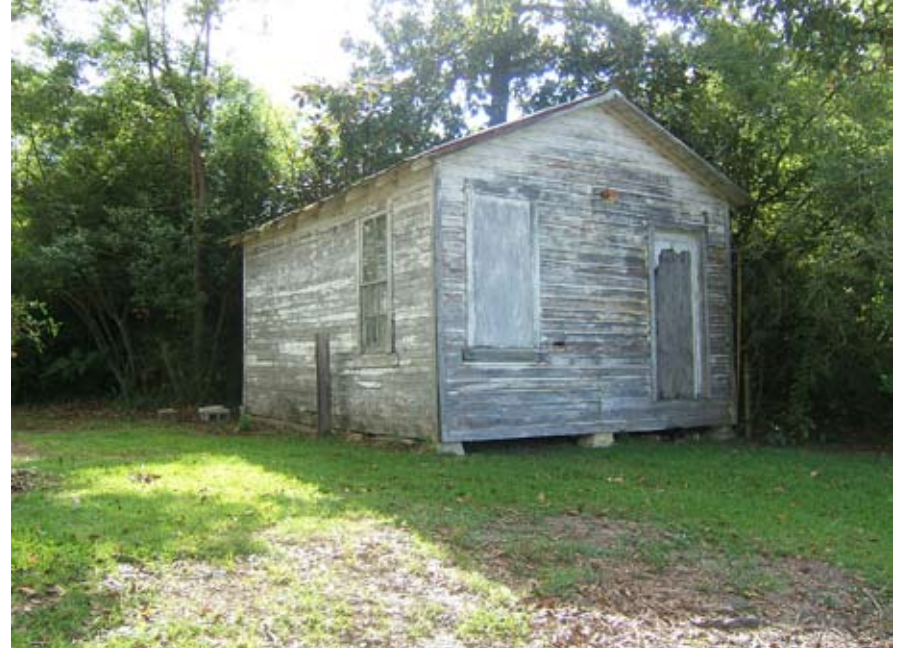
Figure A-14. The historic Lyman Post Office
