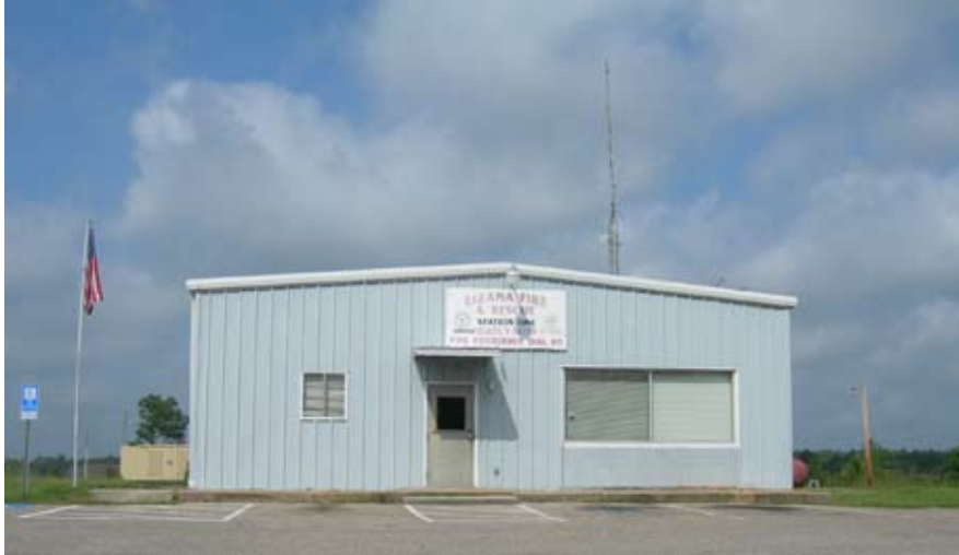
Figure A-34. This fire station serves the Lizana Community
