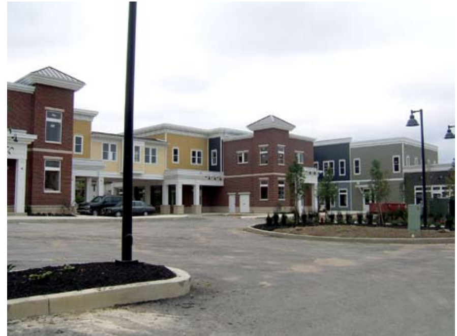
Figure 2-12. This is an example of small scale retail that could be appropriate for the G-3 sector.
