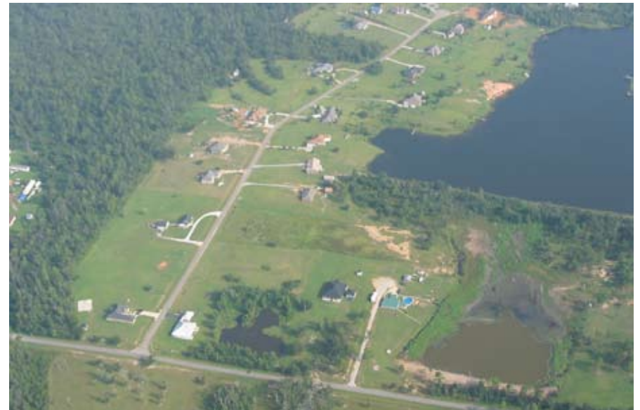
Figure A-22. This residential area is an example of an area zoned as R-1.
