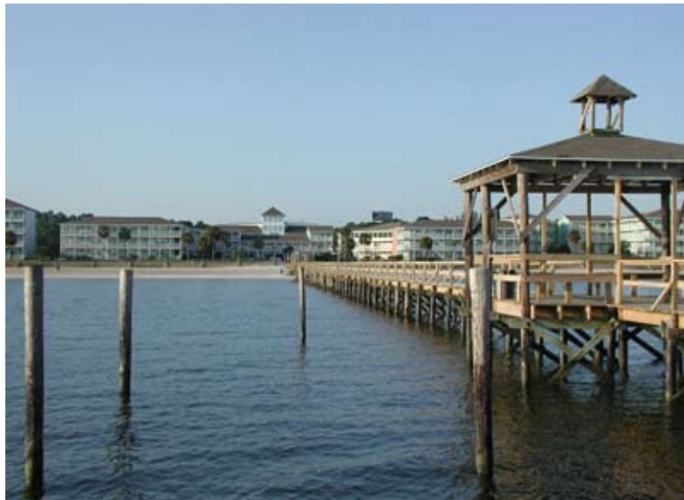
Figure 14. The Village at Henderson Point, which had 70 condominium units, plans to return to the community.
