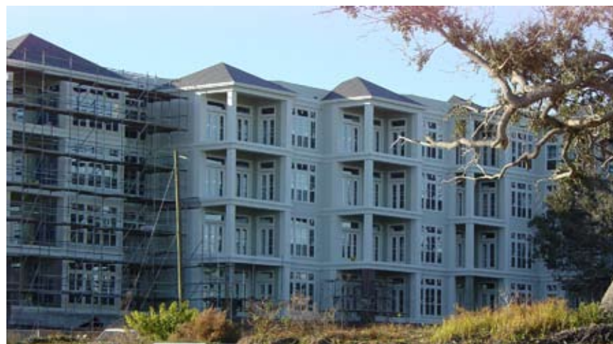
Figure 27. Pass Marianne was under construction at the time of Hurricane Katrina. The project is expected to be complete in 2007.
