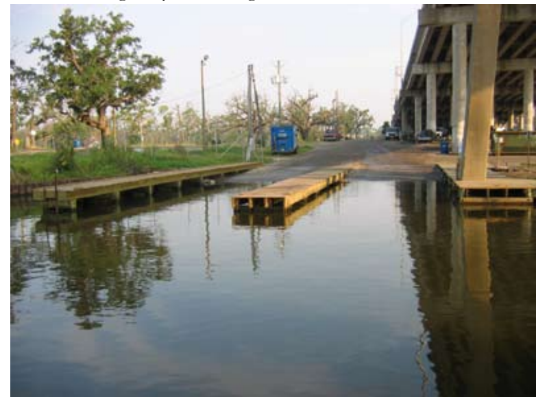
Figure 35. D'Iberville has a boat launch located under the Interstate Highway 110 bridge.
