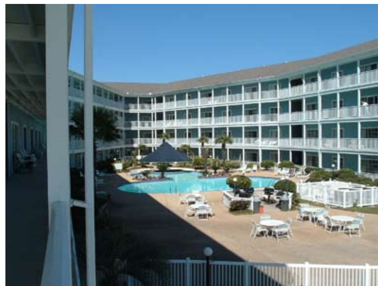
Figure 26. The Inn-by-the-Sea plans to rebuild with the same number of units and same configuration as before Hurricane Katrina.
