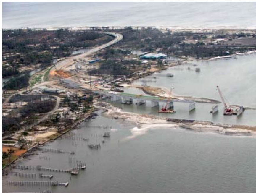
Figure 1. The Henderson Point-Pass Christian community is committed to rebuilding. This photo illustrates the new US Highway 90 bridge under construction.
