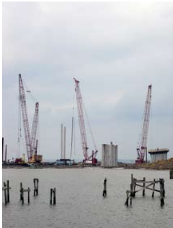
Figure 18. Rebuilding moves forward on the US Highway 90 bridge.
