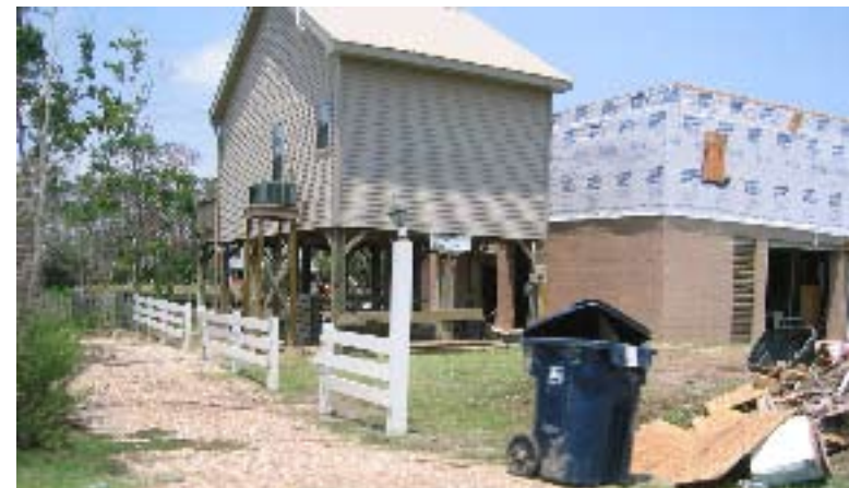
Figure 71. Some of the homes in Henderson Point-Pass Christian Isles are being rebuilt.
