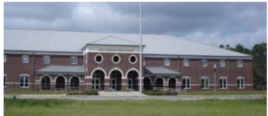
Figure 66. Pass Christian High School underwent repairs following Hurricane Katrina.
