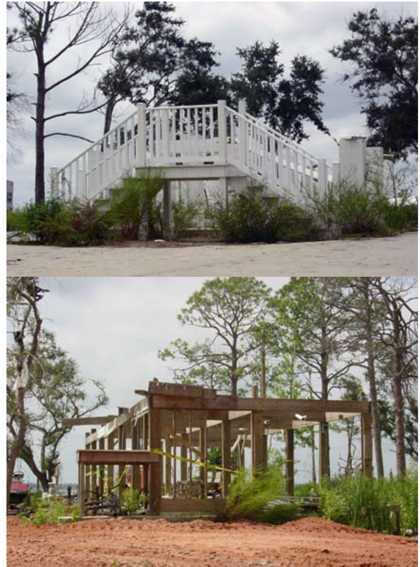
Figure 72. Many homes were elevated before Hurricane Katrina. The ABFE recommendations would require homeowners to elevate higher than before the storm, as shown in these images.
