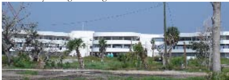
Figure 44. The Gulfshore Baptist Assembly's main building was severely damaged during Hurricane Katrina.
