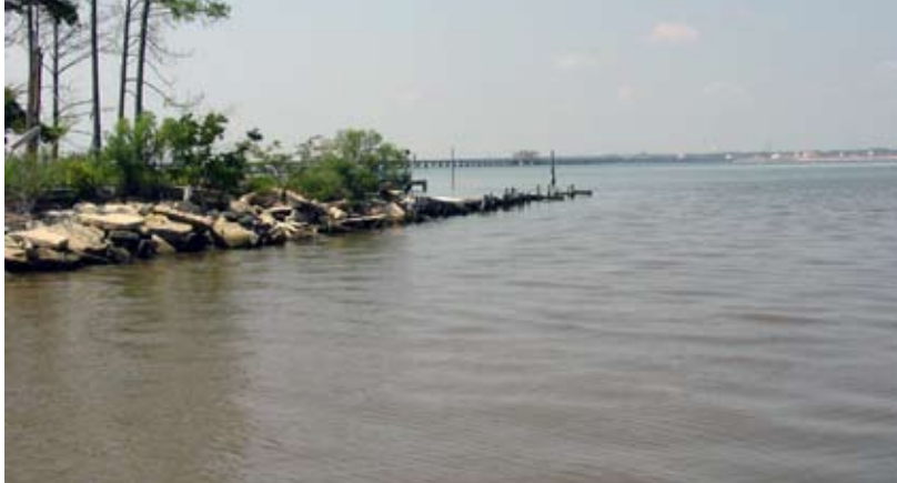
Figure 28. Bayou Mallini connects to the St. Louis Bay.
