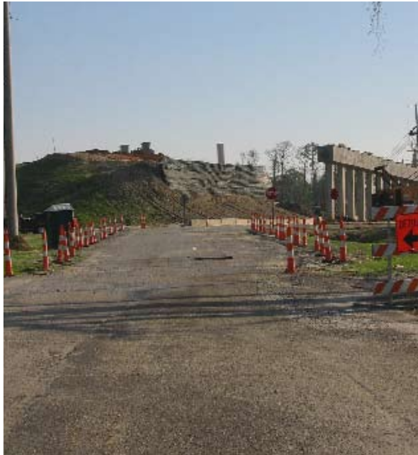
Figure 70. The new US Highway 90 bridge will pass over 3rd Avenue.
