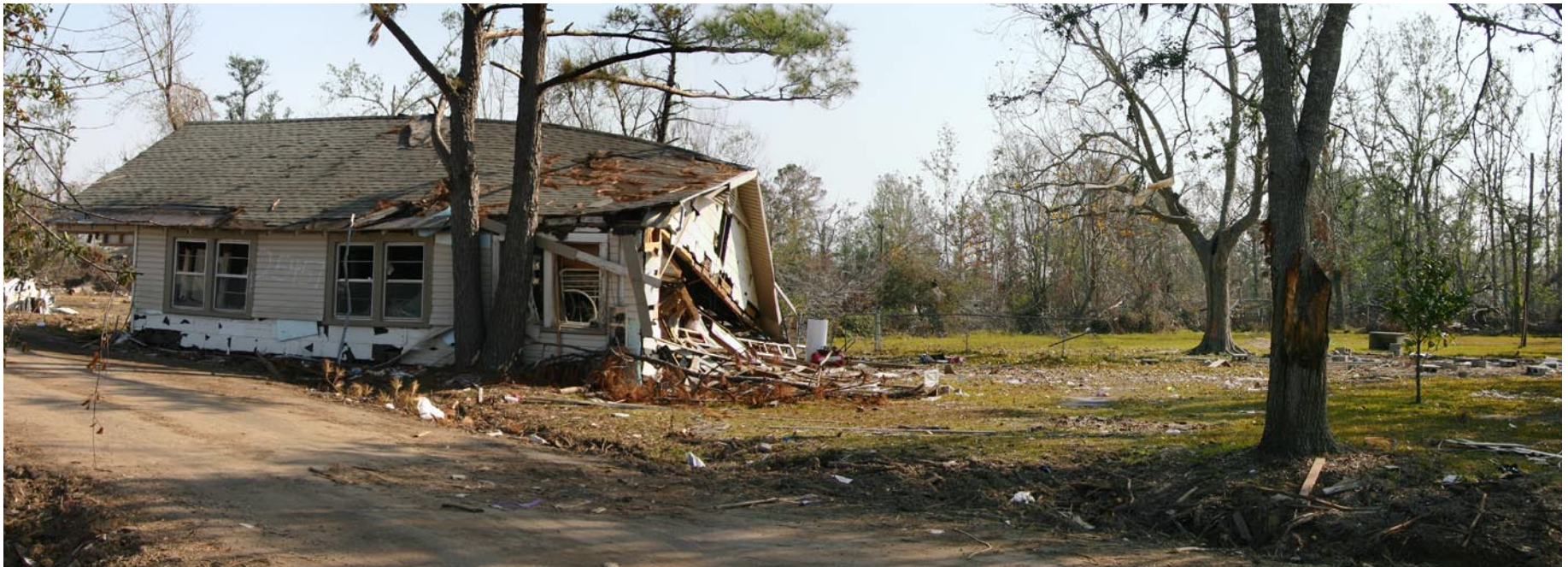
Figure 3 (Bottom). Hurricane Katrina disrupted the lives of DeLisle citizens through its destructive power. The storm's surge pushed this house near Bayou DeLisle off of its foundation. Source: Michael Curtis.
