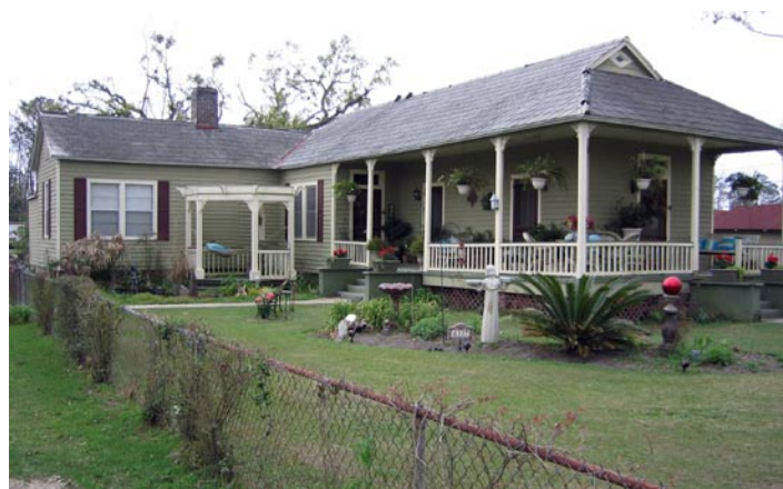
Figure 52: One of the oldest houses in the DeLisle is still standing after Hurricane Katrina.
