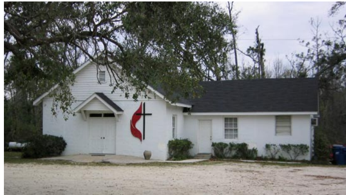
Figure 47. Mt. Zion United Methodist Church located on Lobouy Road was last updated in the 1960s. A new church is being built on Kiln-DeLisle Road and will accompany housing units and a community center. Source: Michael Curtis.
