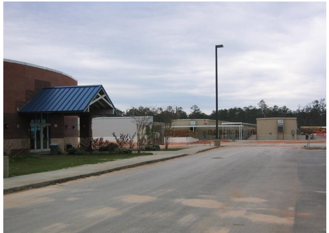
Figure 46. DeLisle Elementary School post-Katrina. The trailers on the property function as classrooms and school district administrative offices.
