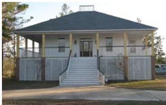
Figure 21 (Top). A house raised on masonry piles.
