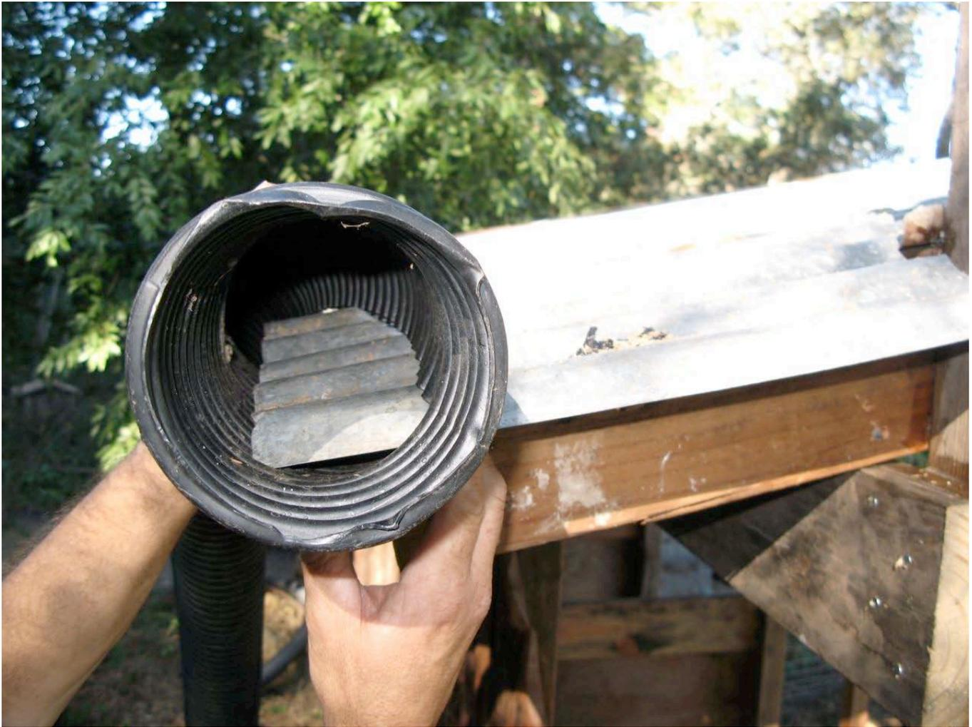
Here you can see the cross section of the pipe over the edge of the roofing. We made sure to let the roofing overhang about 3-5" to allow space for the drainpipe to slide over the edge. Here you can see how we left the first four inches uncut to allow for an end cap.
