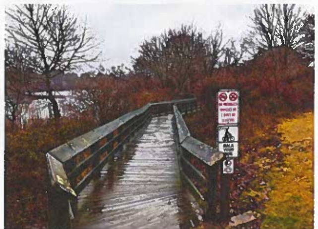
Poquonnock River Boardwalk
