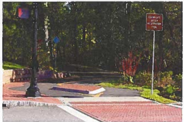
Median island path access, Source: Weston & Sampson
