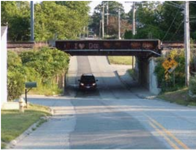
South Road underpass
